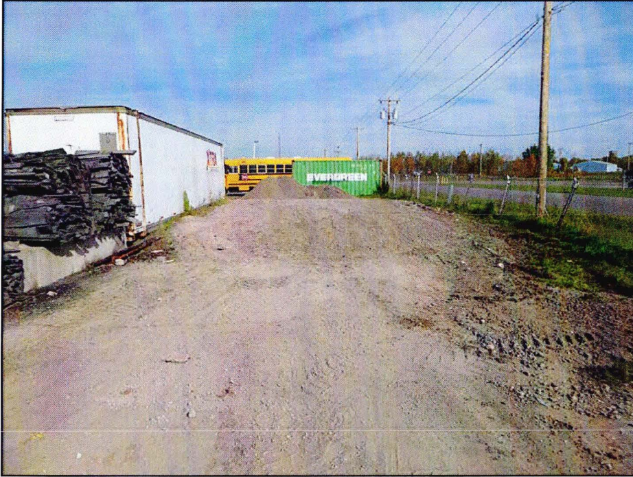
Surface restoration following abandonment
