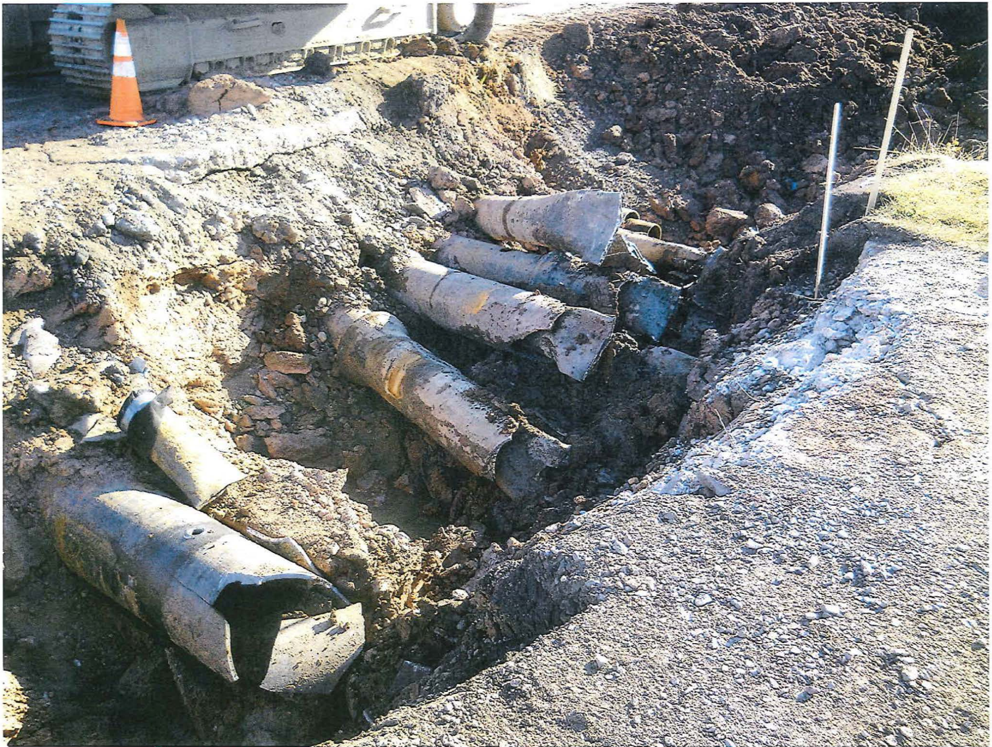
Petro Lines 112+50 (Antea Entrance) Pipe Removals
