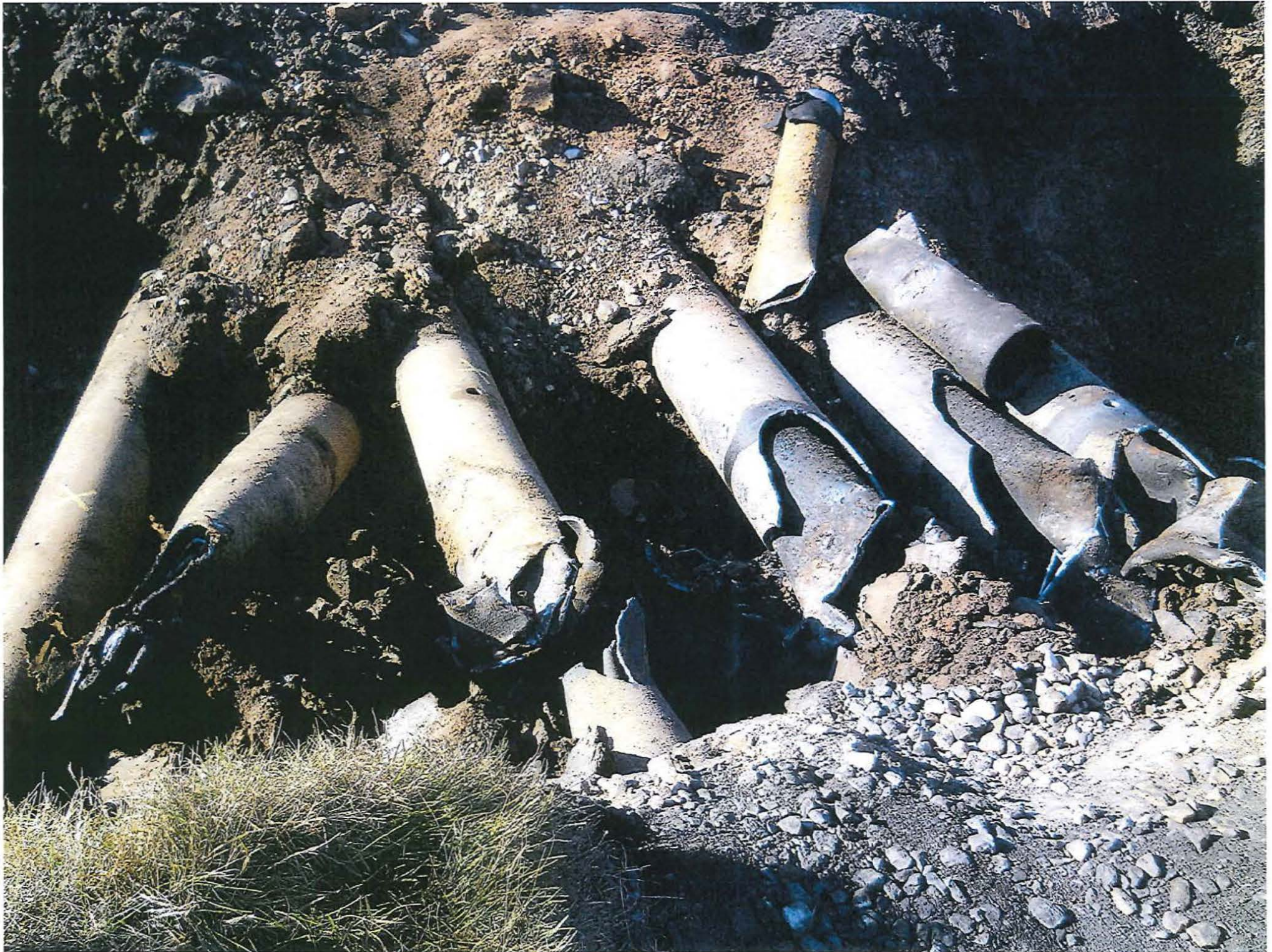
Petro Lines 112+50 (Antea Entrance) Pipe Removals
