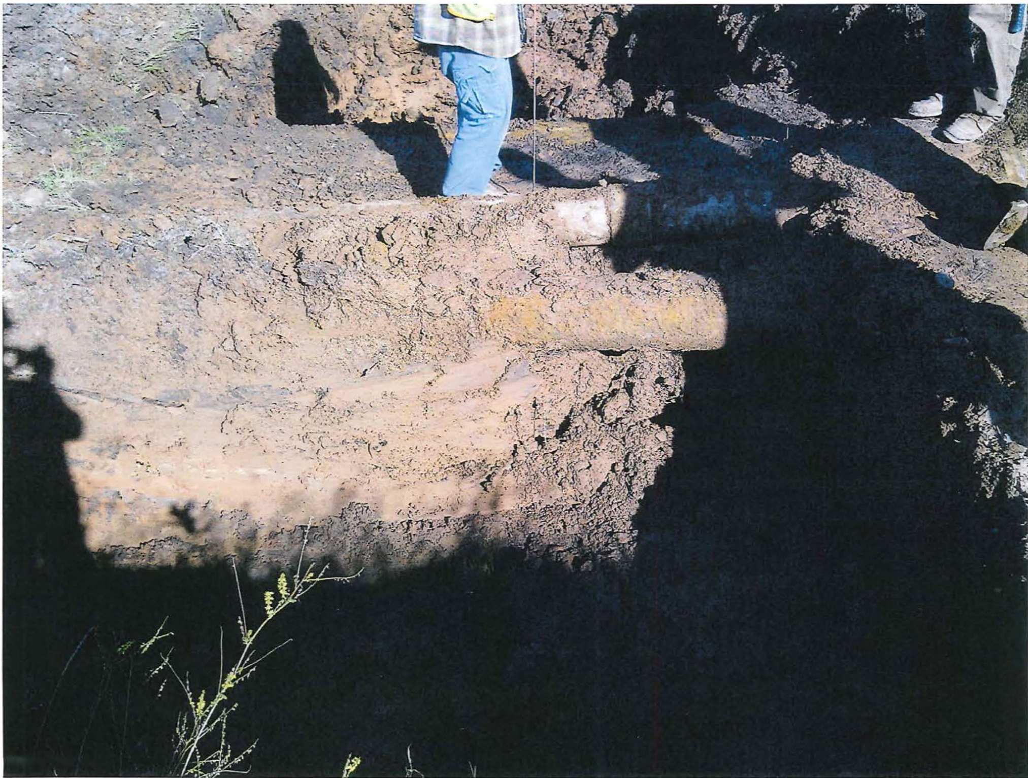
Locate Petro Lines 112+50 (Antea Entrance)
