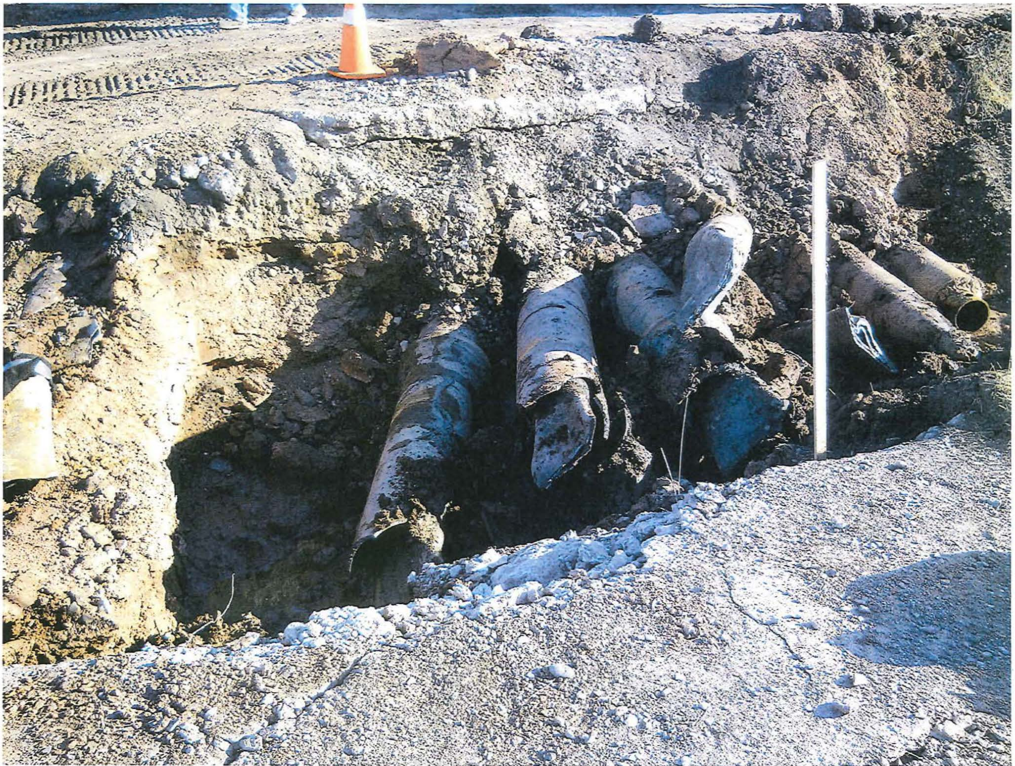
Petro Lines 112+50 (Antea Entrance) Pipe Removals
