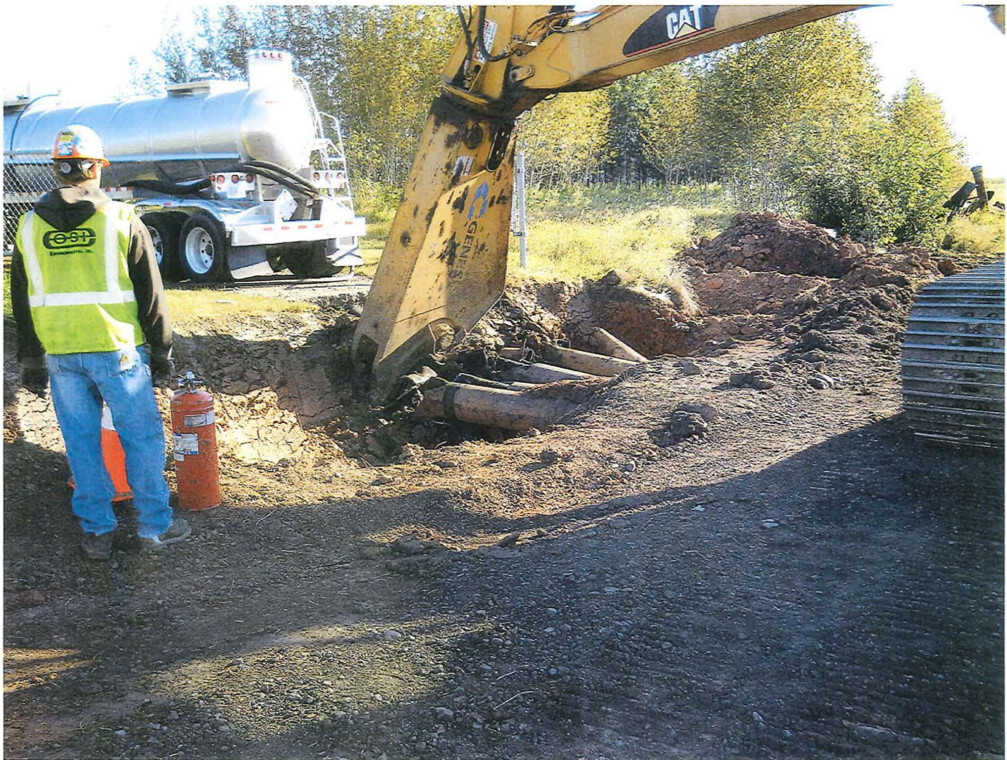
Petro Lines 112+50 (Antea Entrance) Pipe Removals
