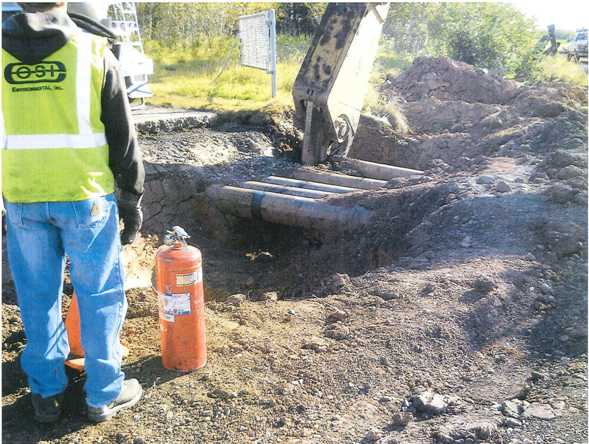
Petro Pipes 112+50 (Antea Entrance) Pipe Removals
