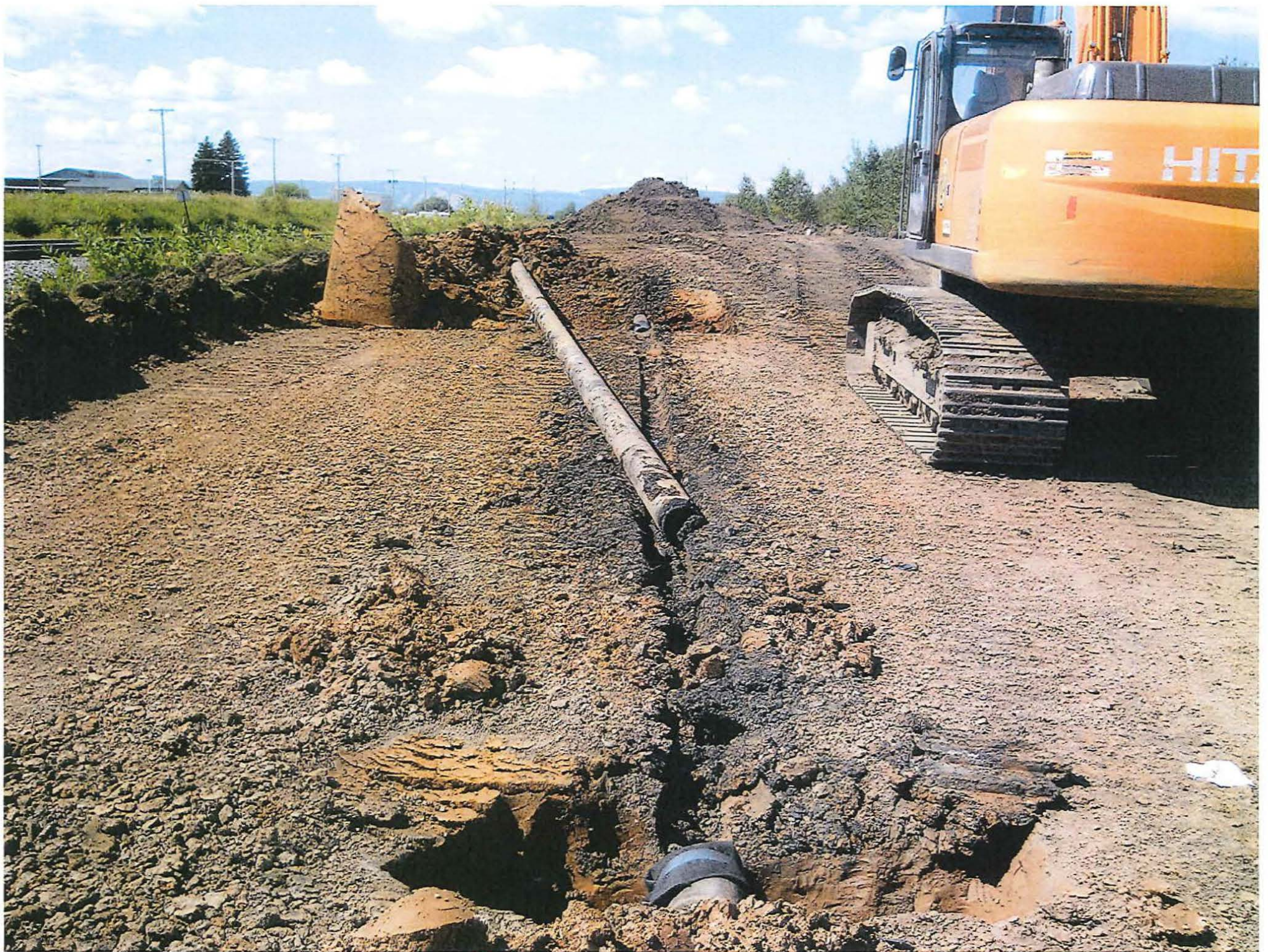
Aband. Petro Line in Rd. Subgrade 105+25 to 106+25±
