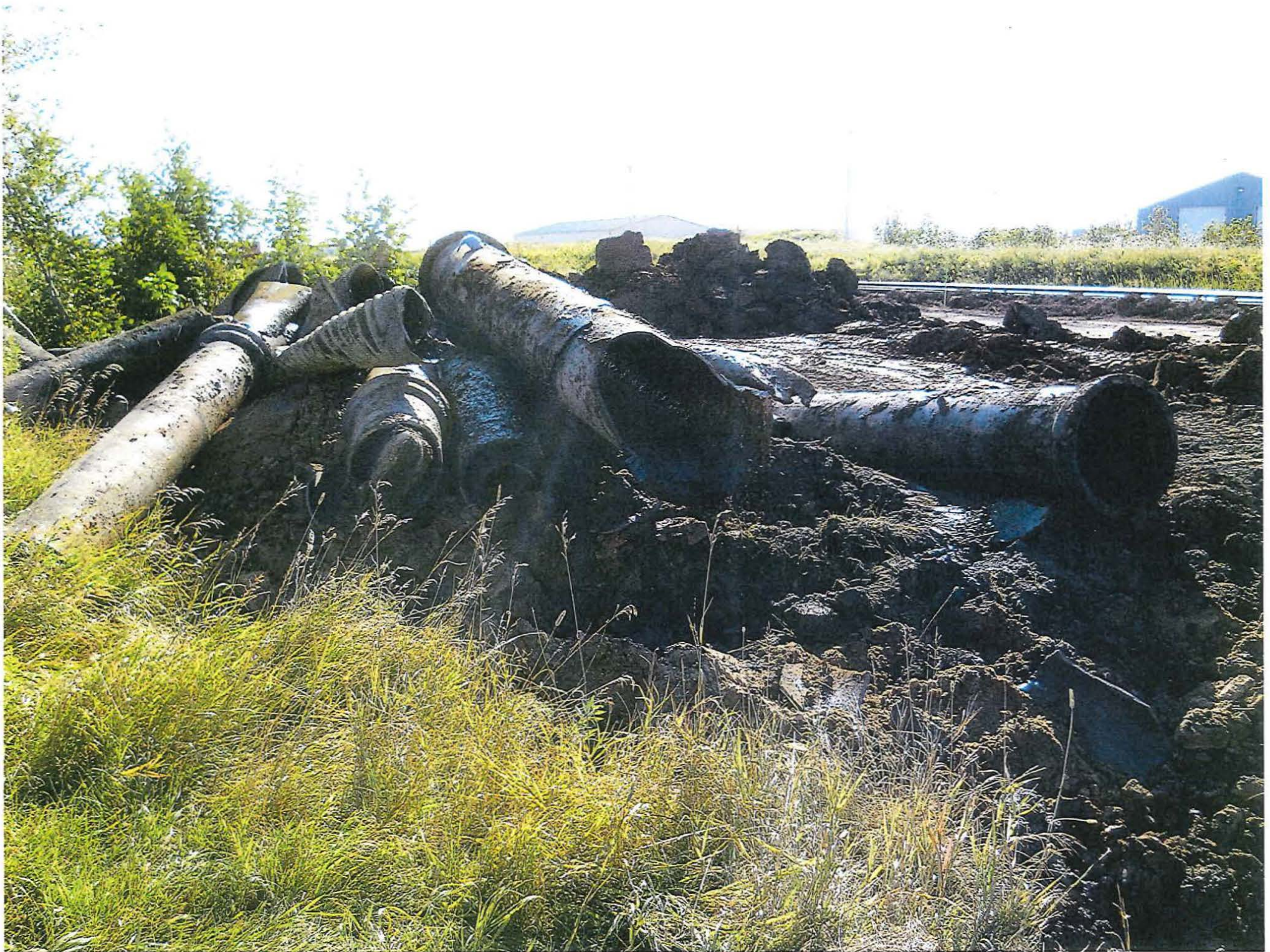
Petro Lines 112+50 (Antea Entrance) Pipe Removals
