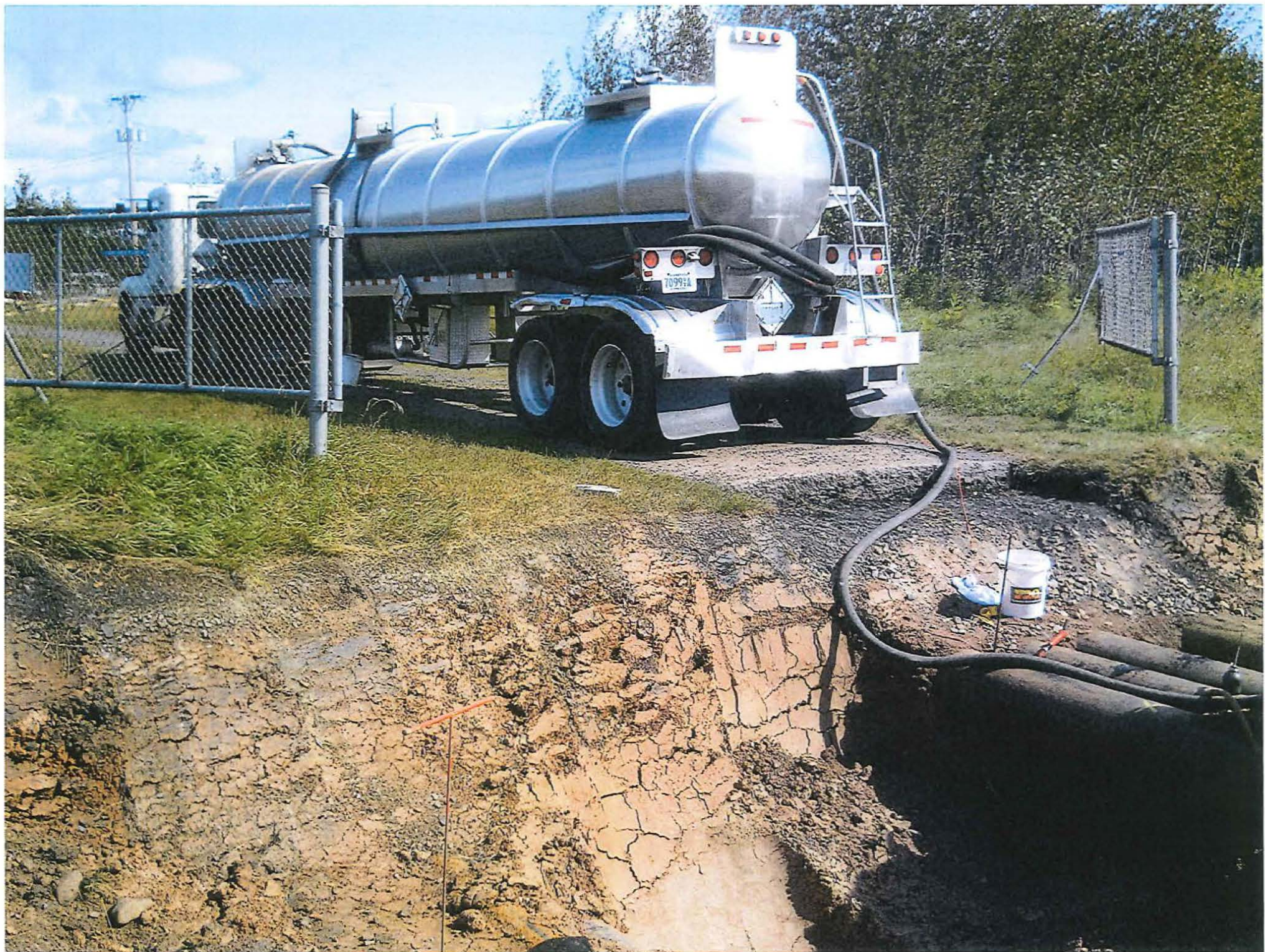
Petra LWB3 112+50 (Antea Entrance) Residue Removal / Investigation
