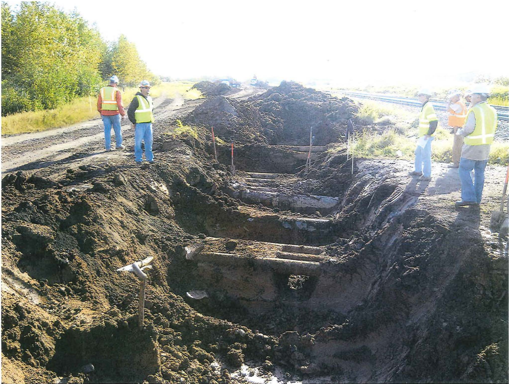
Locate Petro Lines 112+50 (Antea Entrance)
