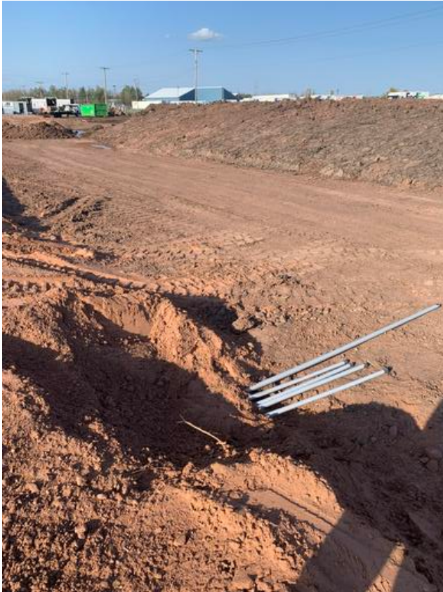
Conduit Extensions @ East Van Lot
