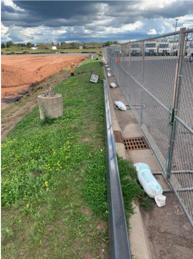
Disconnect & salvage light poles @ east lot
