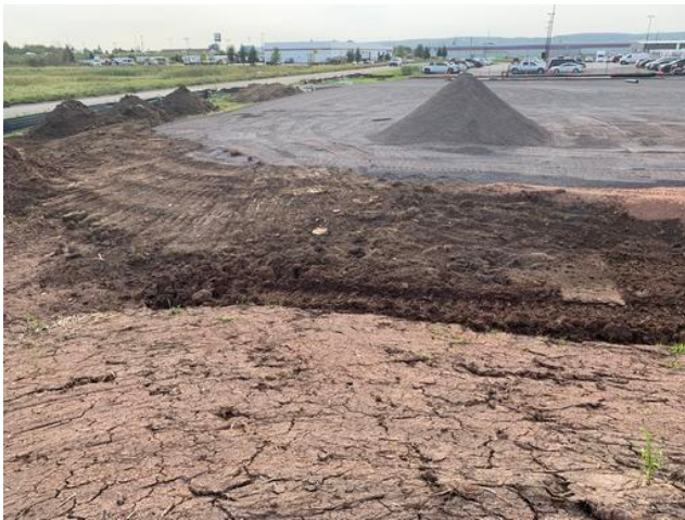
Shoulder employee lot with top soil
