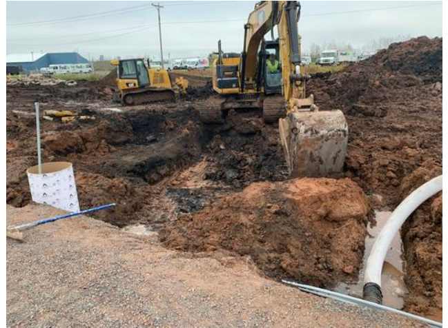
Excavating pond and removing debris Scott Luostari Oct 5, 2021 4:10 PM
