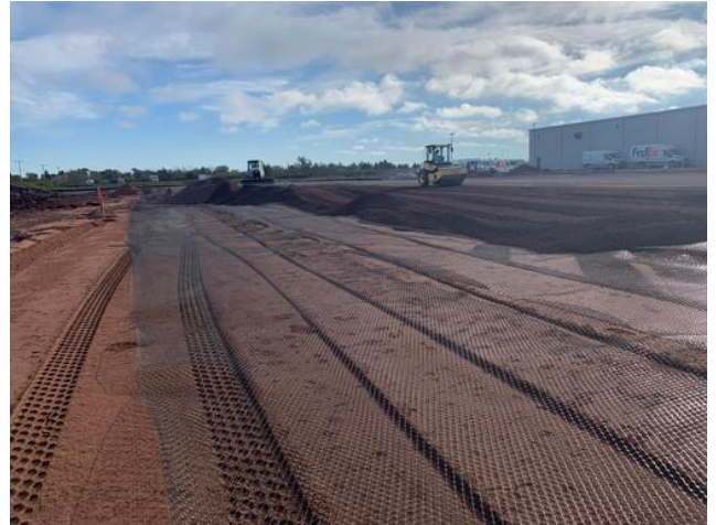
Geogrid and Gravel Placement on Van Lot
