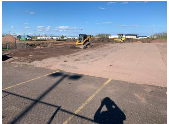
Rough Grade Employee Lot
