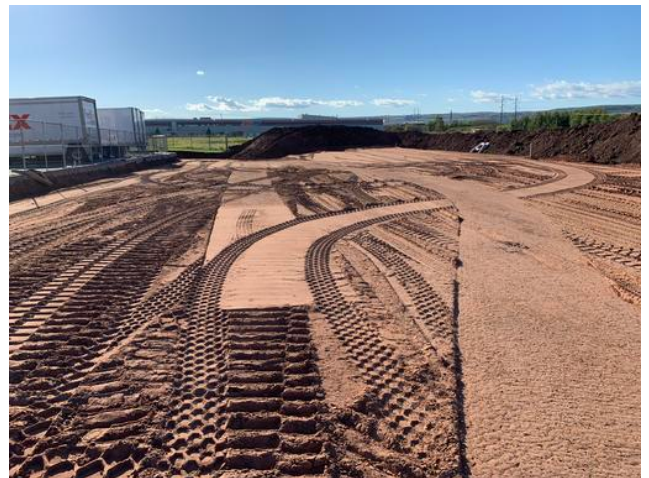
Sand Placement on West Trailer Lot
