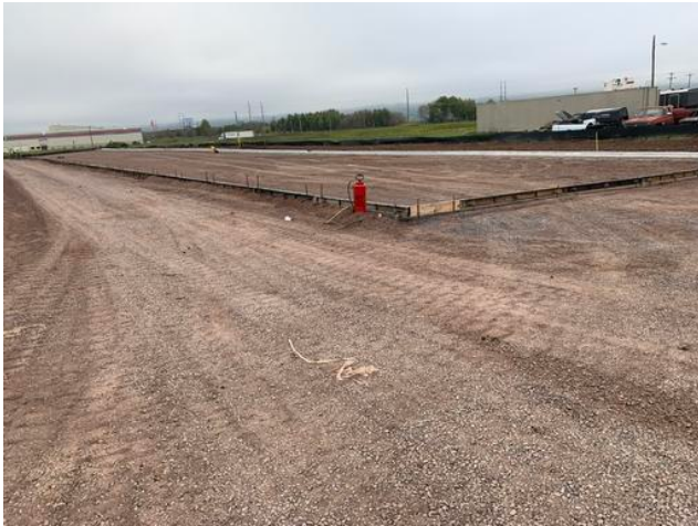
Trailer paving formed Scott Luostari Oct 5, 2021 4:10 PM
