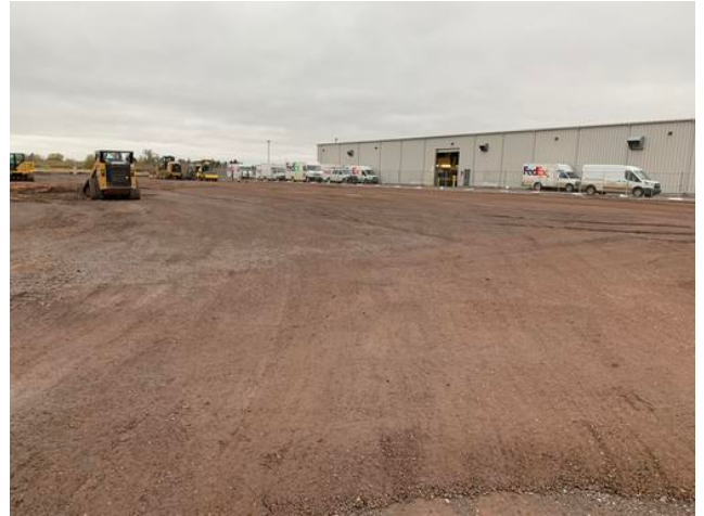
Fine Grading of Van Lot
