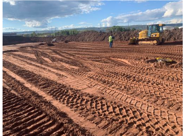
Sand Placement on Trailer Lot
