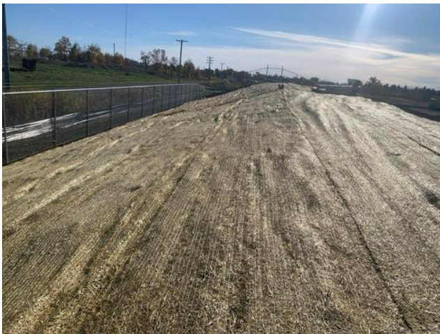
E-Mat and Fencing on Berm
