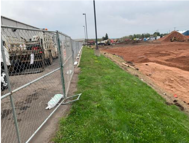
Existing Fence Removal
