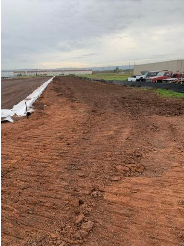
Grading North of Trailer Paving Curb
