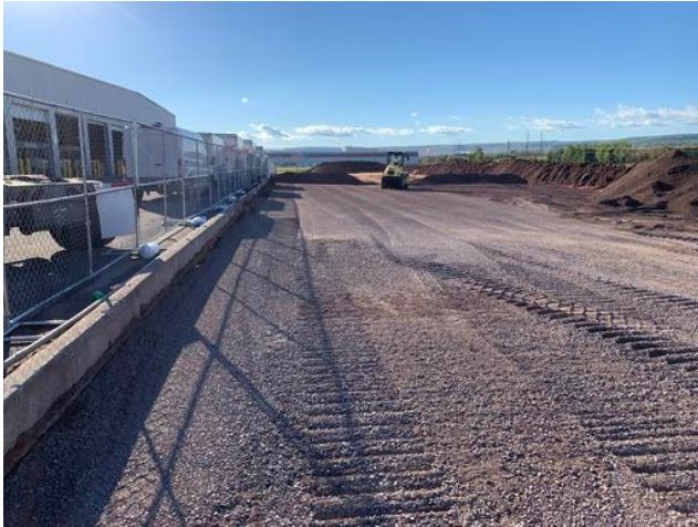
GeoGrid and Gravel on Trailer Lot
