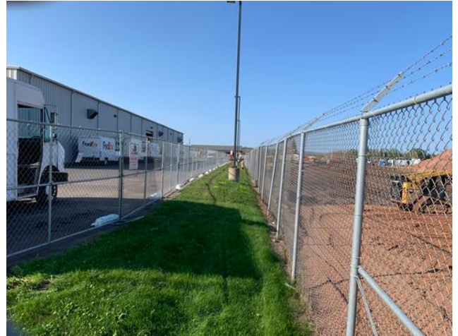
Temp Fence Install
