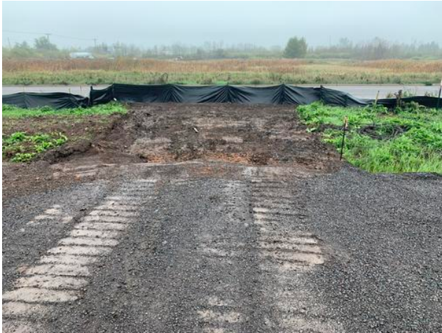
South Entrance Removed
