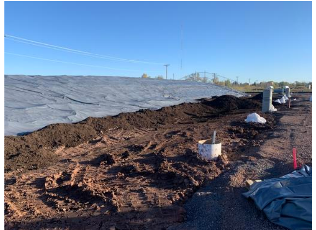
Berm PVC Liner
