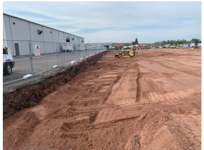
Sub-cut and import sand east lot transition
