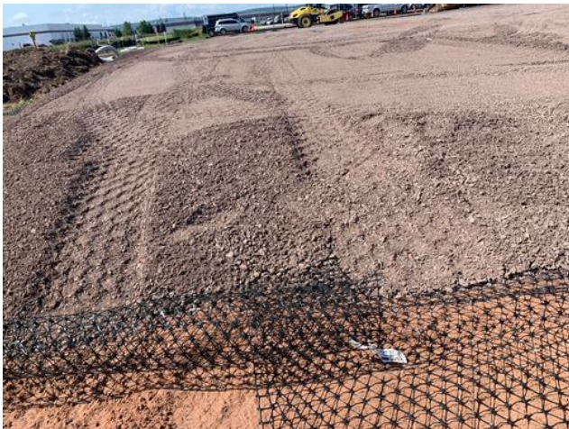
GeoGrid and Gravel
