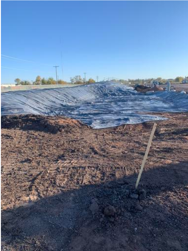
Pond & Berm PVC Liner
