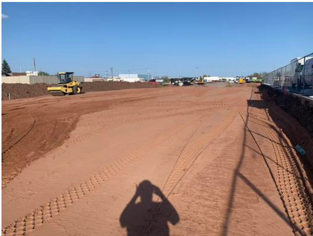
Sand Compaction @ Trailer Lot
