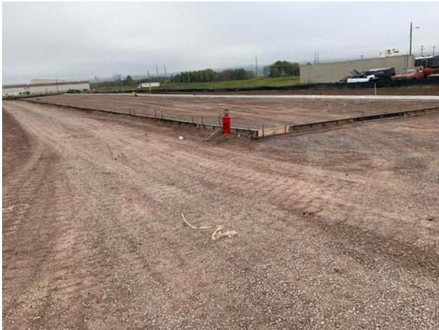
Trailer paving formed
