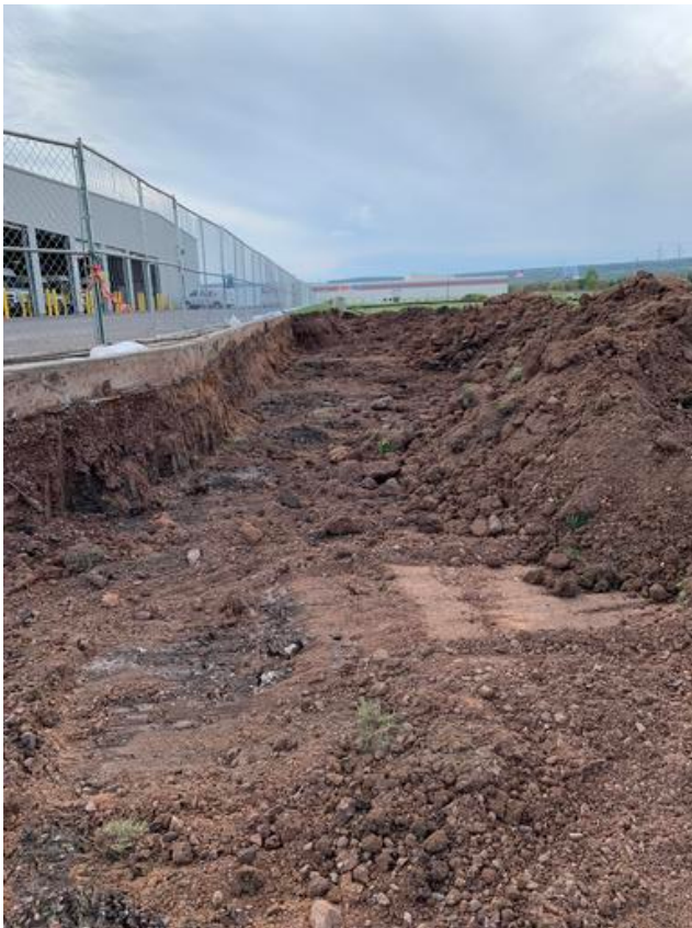
Sub-Cutting Trailer Lot
