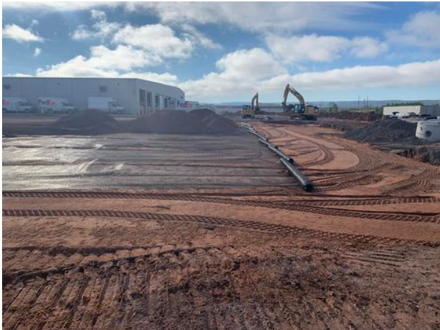
Geogrid & Gravel at NE Corner of Site
