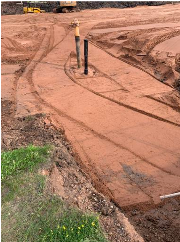
Fire hydrant relocation
