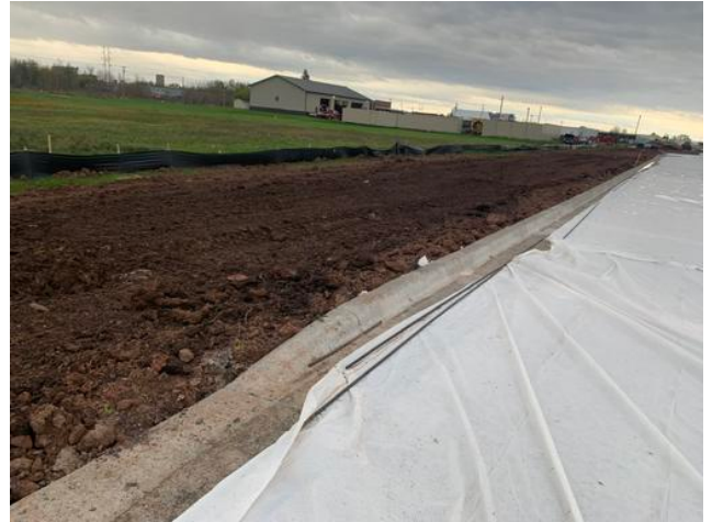
North Site Perimeter Grading
