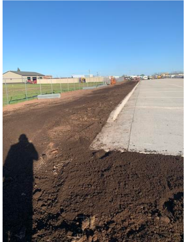
Fence & Topsoil at N Edge of Trailer Lot
