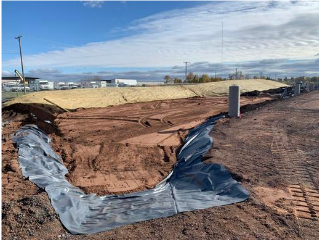
Liner & Sand in Pond Scott Luostari Oct 22, 2021 2:09 PM
