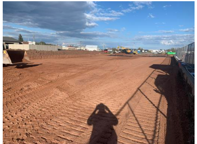
Fine Grading of Sand on Trailer Lot
