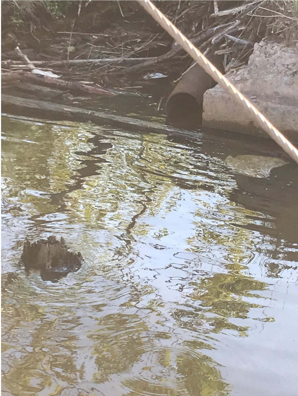
Pipe (possible outfall) next to concrete at the head of the Amoco Barge Slip, Superior Wi. Viewing south. Taken July 2, 2022, by Joe Graham.
