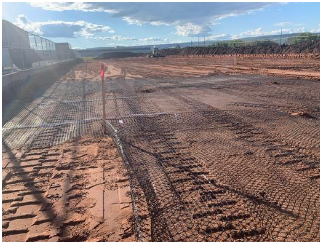
GeoGrid on Trailer Lot
