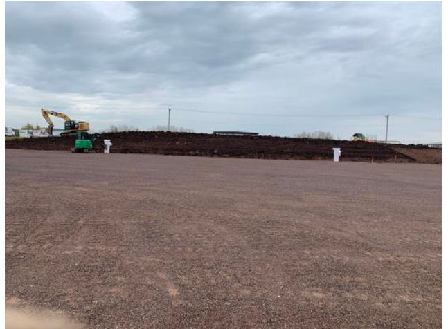
Light Pole Foundations & Berm Shaping
