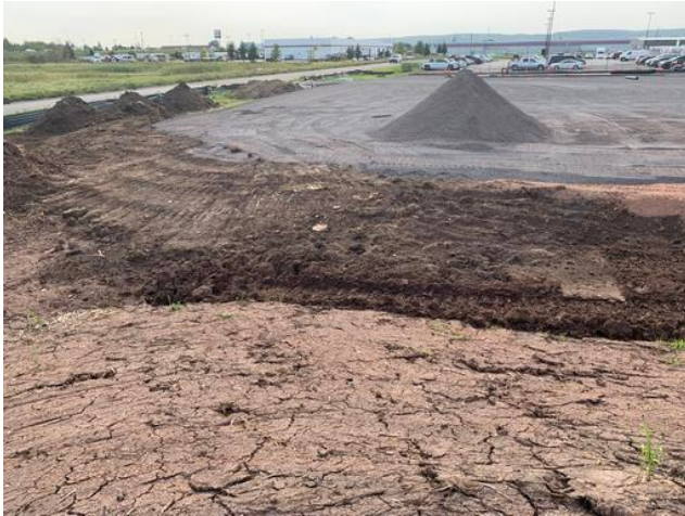
Shoulder employee lot with top soil
