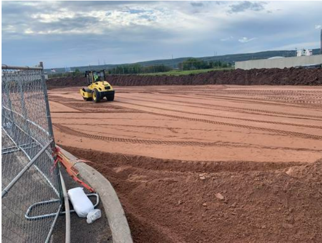
Compacting Sand on Trailer Lot
