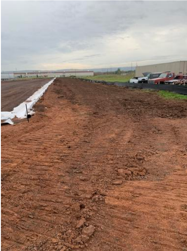
Grading North of Trailer Paving Curb
