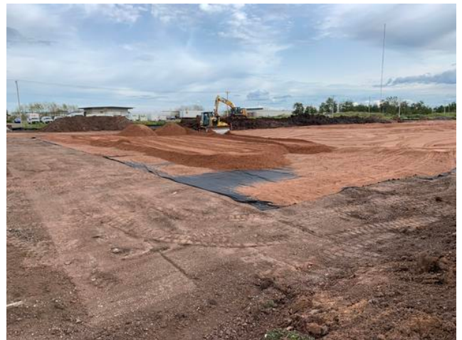
Import and grade sand at north end of van lot
