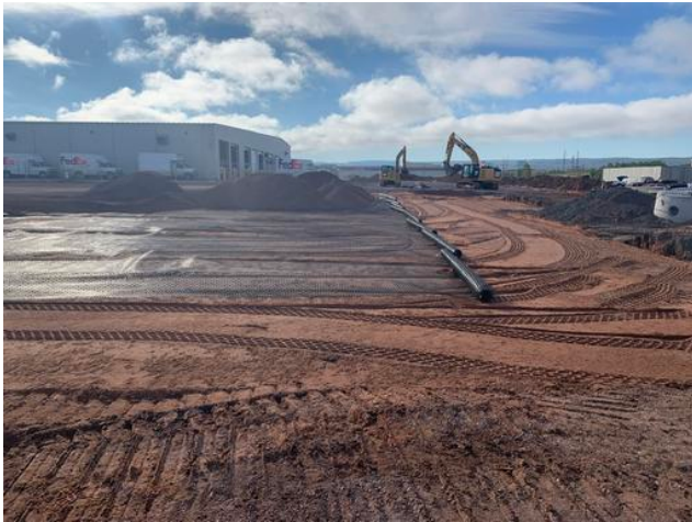
Geogrid & Gravel at NE Corner of Site
