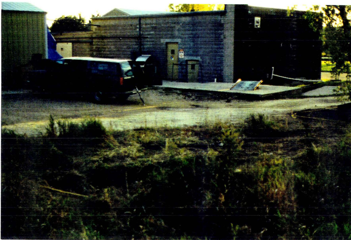
PHOTOGRAPH #4: LOOKING SOUTHWEST AT SAMPLE LOCATIONS 10 - 16 IN ORIGINAL TRAILER AREA EXCAVATION
