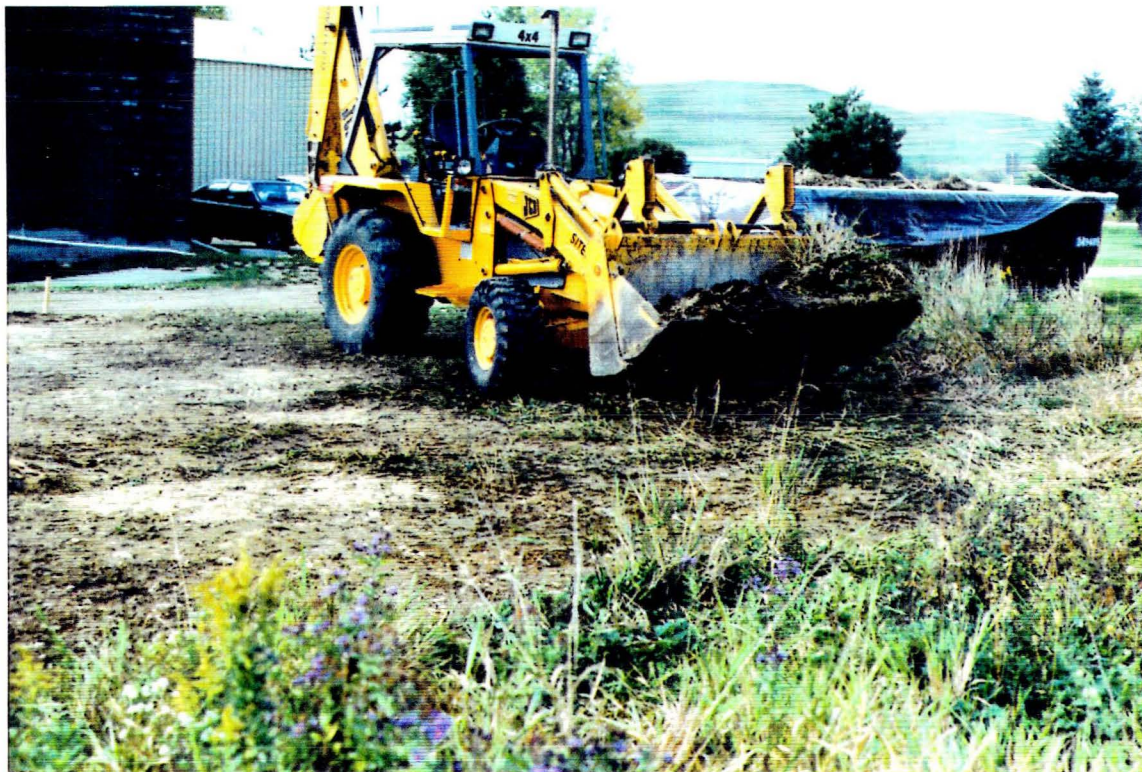
PHOTOGRAPH #2: EXCAVATED SOILS LOADED INTO ROLL-OFF CONTAINERS
