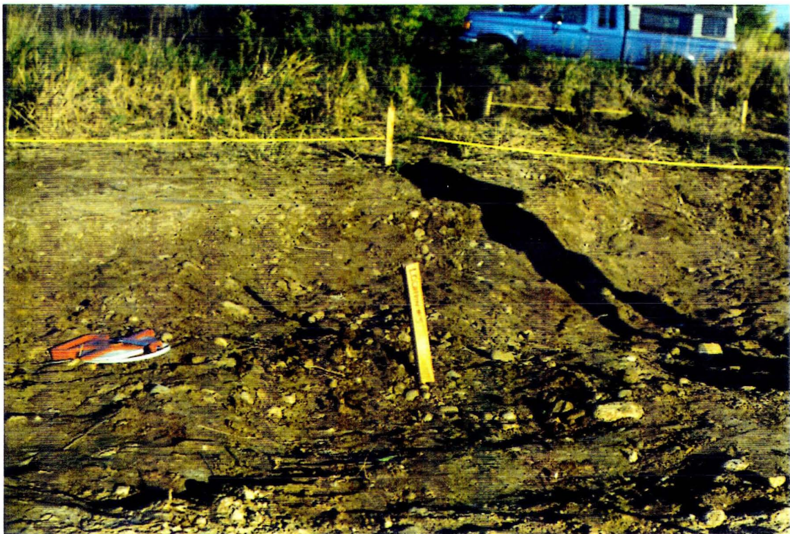
PHOTOGRAPH #6: SAMPLE LOCATION #5 IN AREA OF 6" EXCAVATION
