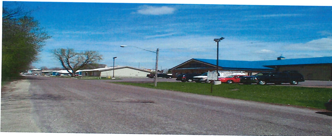
National Auto Wrecking Co., Inc. site Subdivided into four lots for redevelopment 2 nd Avenue SW looking north
