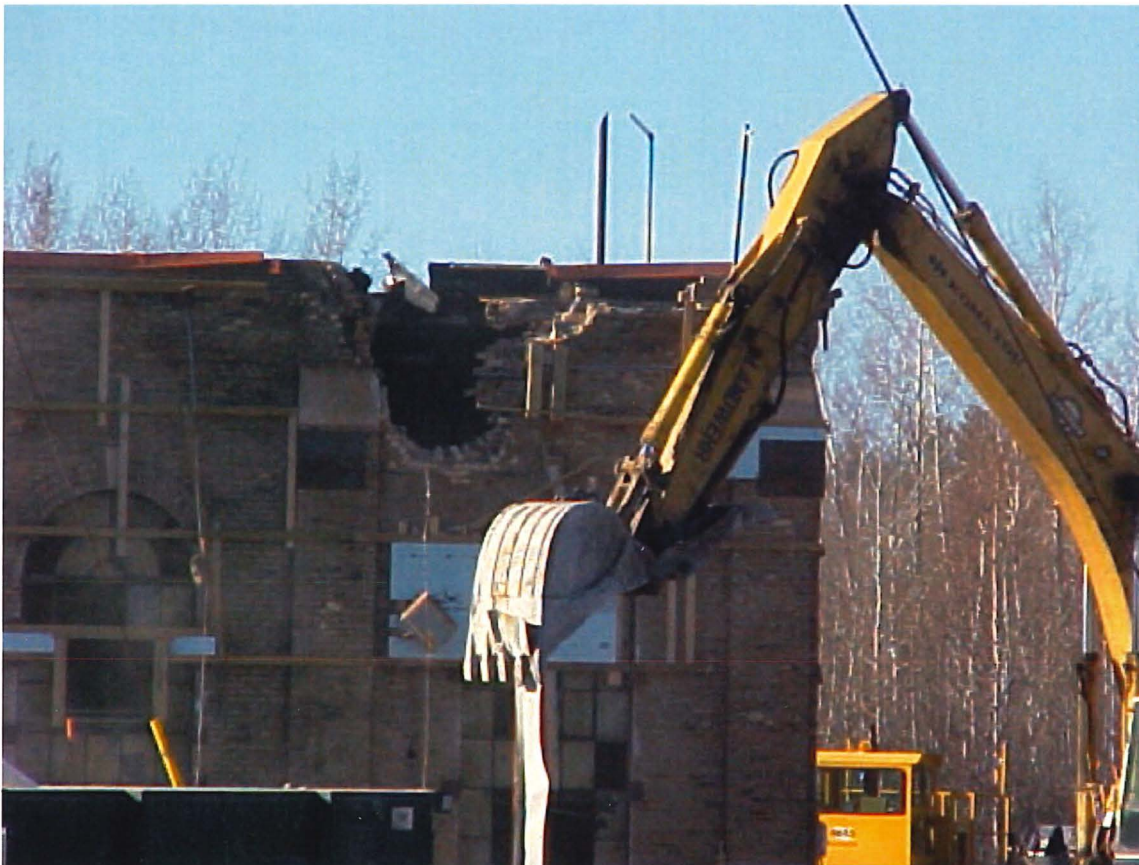
The start of taking down the building.
