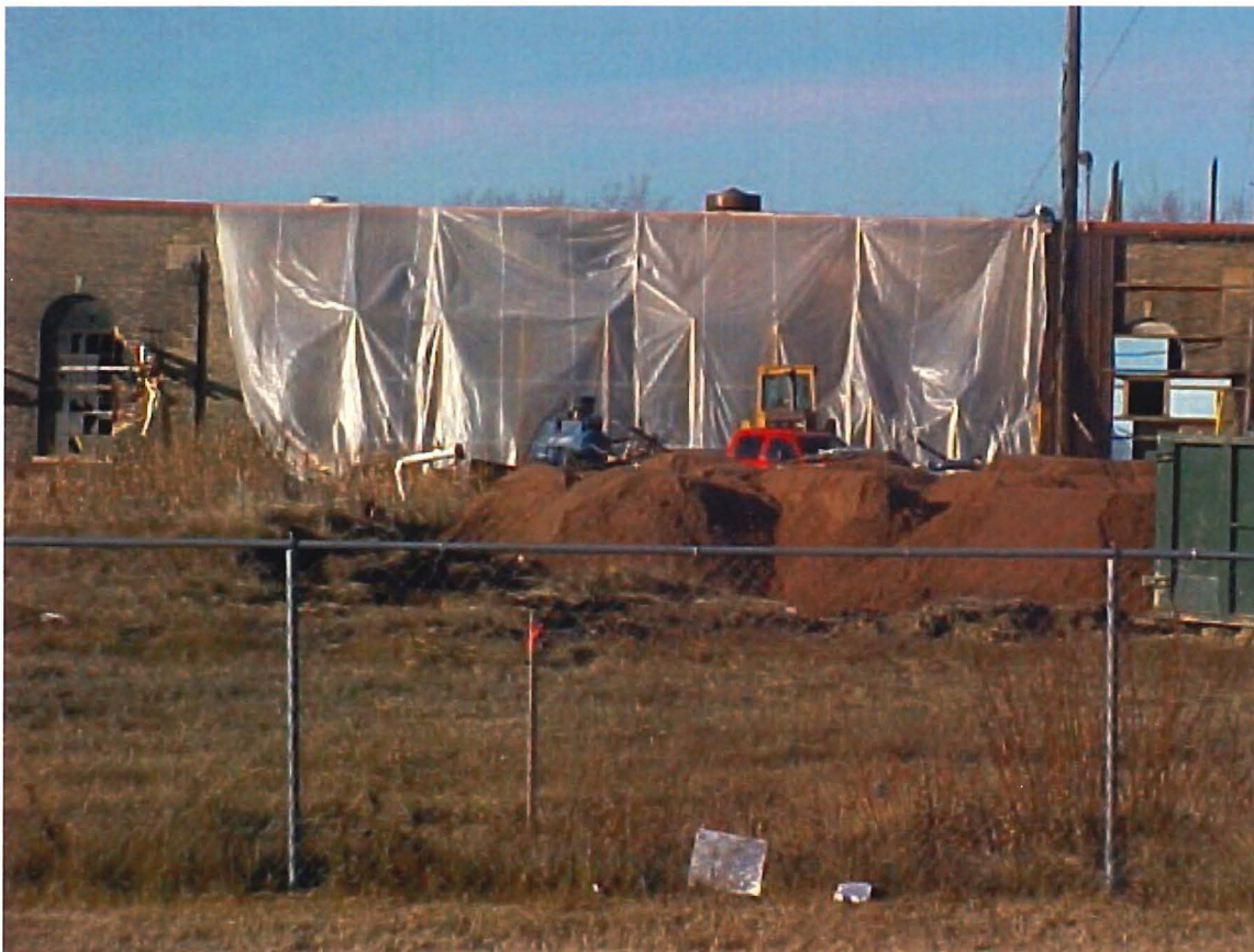
Example of east exterior wall isolated off prior to sandblasting.
