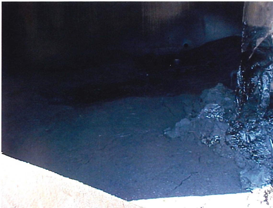
Inside of creosote storage tank prior to cleaning.
