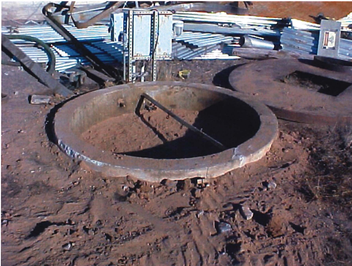
Main sump of drip pad filled with clean sand after pressure washing.
