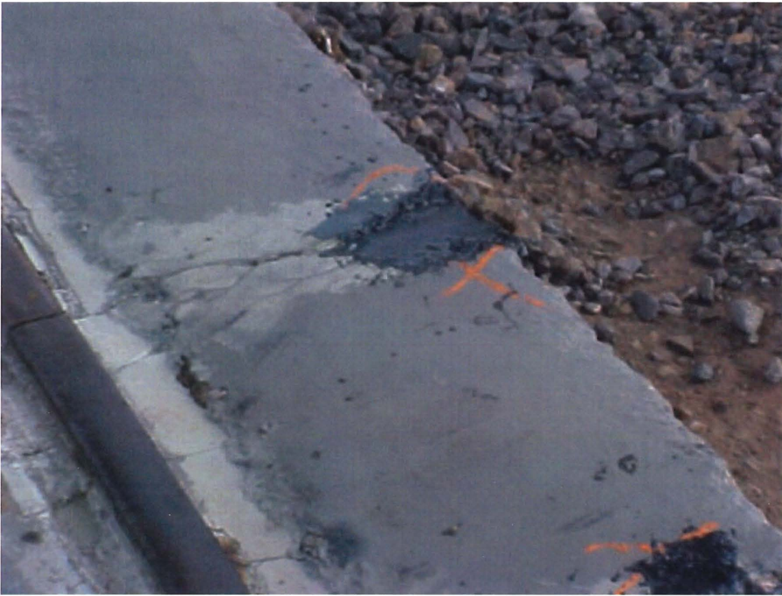
True Bond applied to repair cracks in surface of drip pad.
