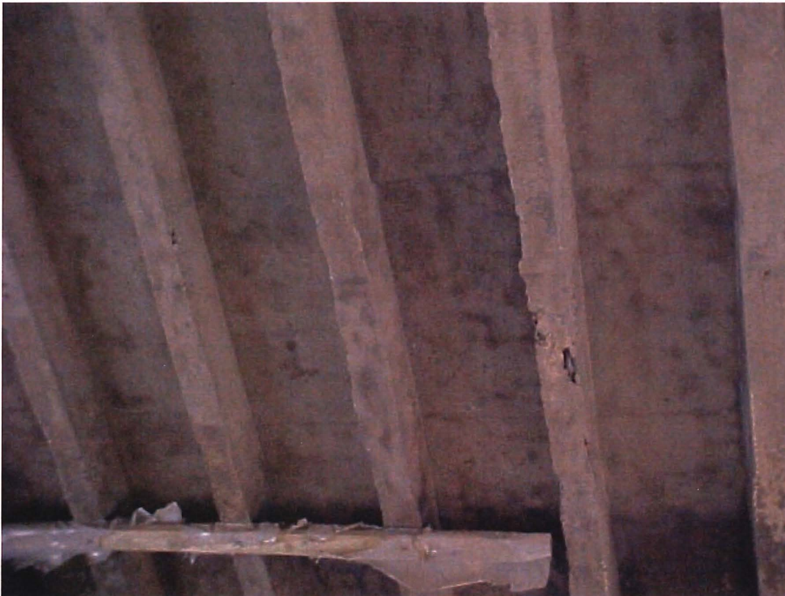
Ceiling above air tank after sandblasting
