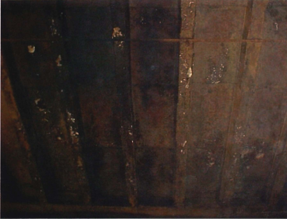
Ceiling above air tank prior to sandblasting
