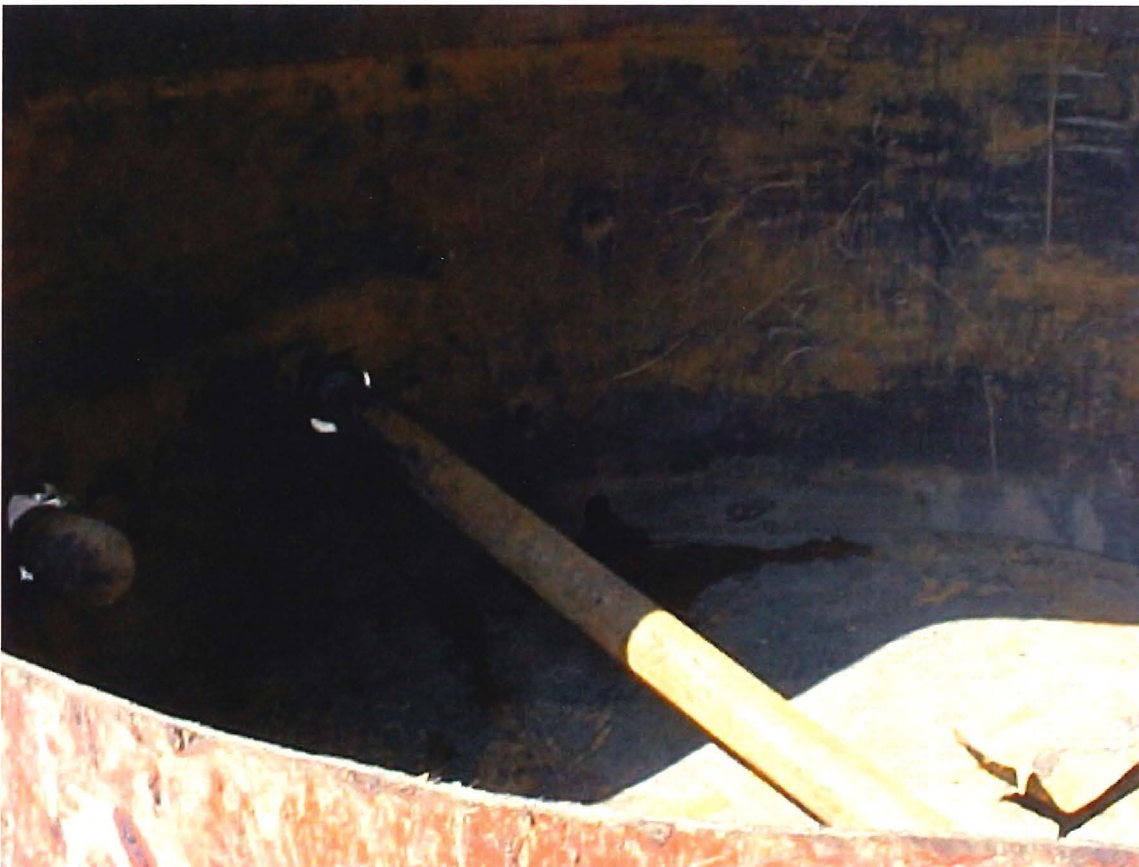
Inside of B tank after cleaning.
