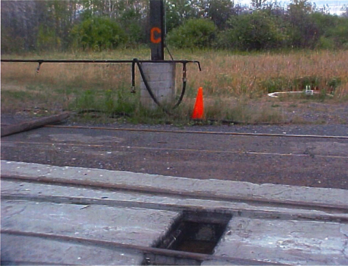
Example of drain line closed off in basin after pressure washing drain line.
