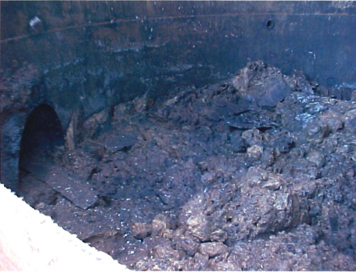
Inside of B tank prior to cleaning.
