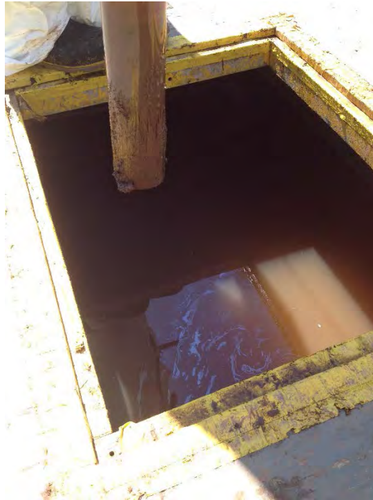
Sheen / NAPL blobs appearing on the water surface at a Crawford Creek sample location
