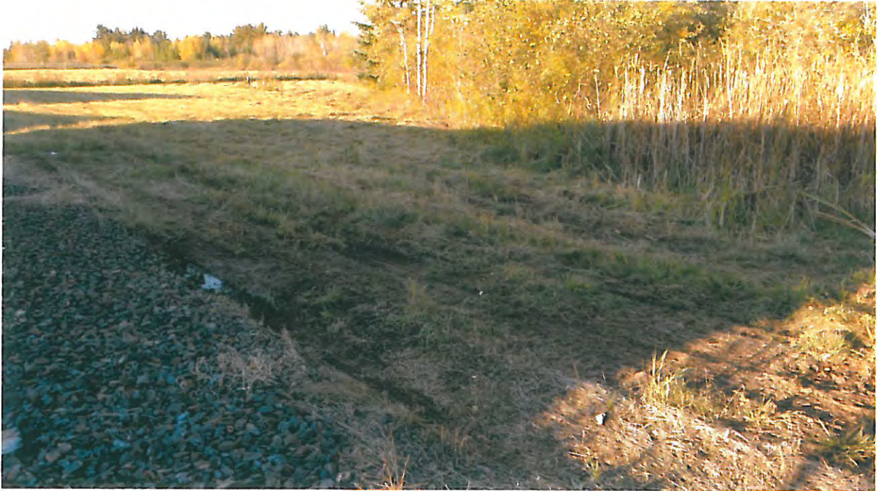
Area B Photo 12, Close up of ruts from Photo 4:
