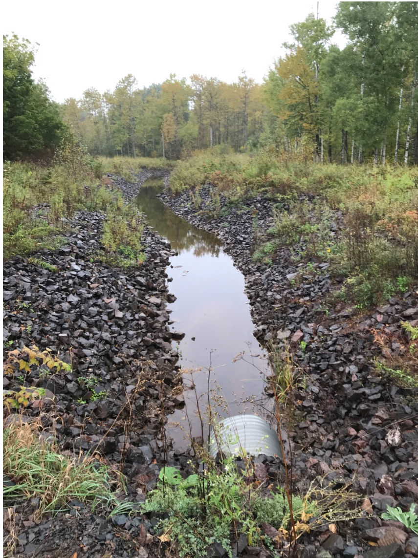
Outfall 001 Drainage Ditch Photo 2, looking west from center:
