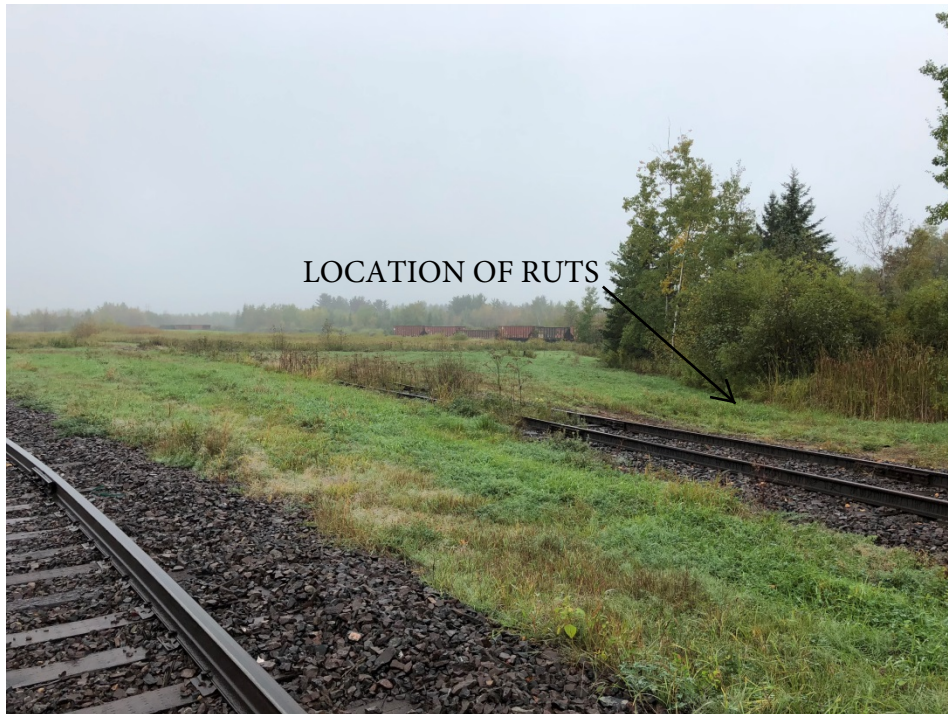
Area B Photo 4, looking South from North West along (ruts in grass along gravel):
