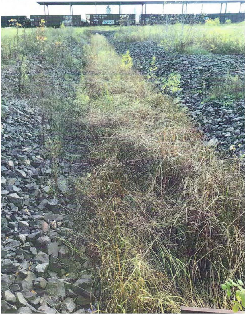
Drainage ditch p2
