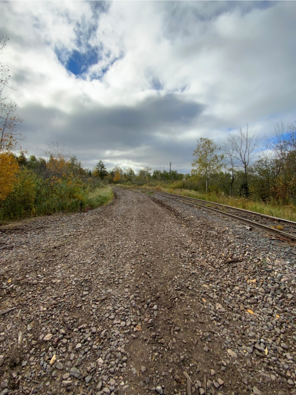
Area H Photo 1, (East side of RR tracks) looking Southwest from Eastern side:
