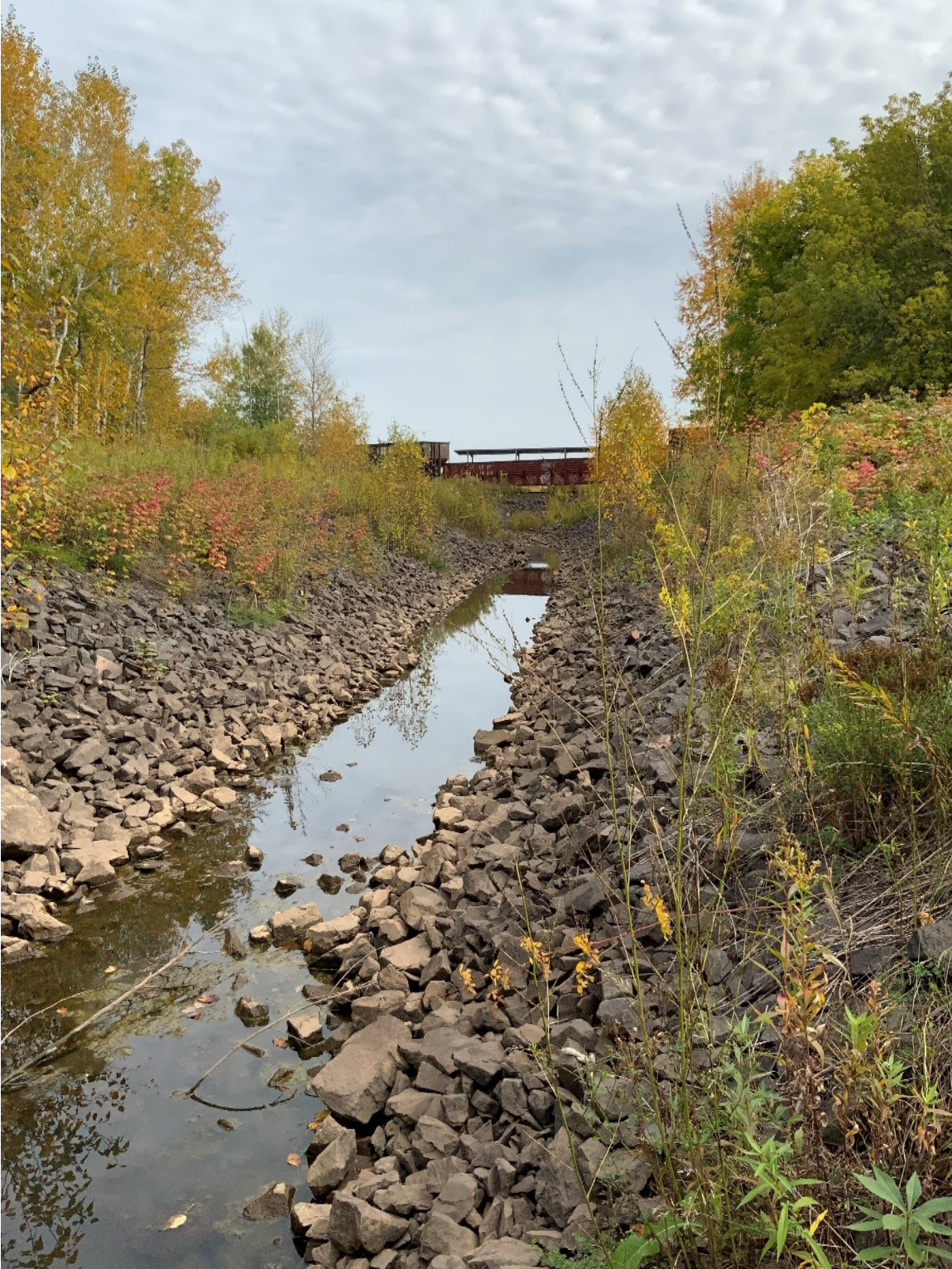
Outfall 001 Drainage Ditch Photo 4, looking East from Western edge:
