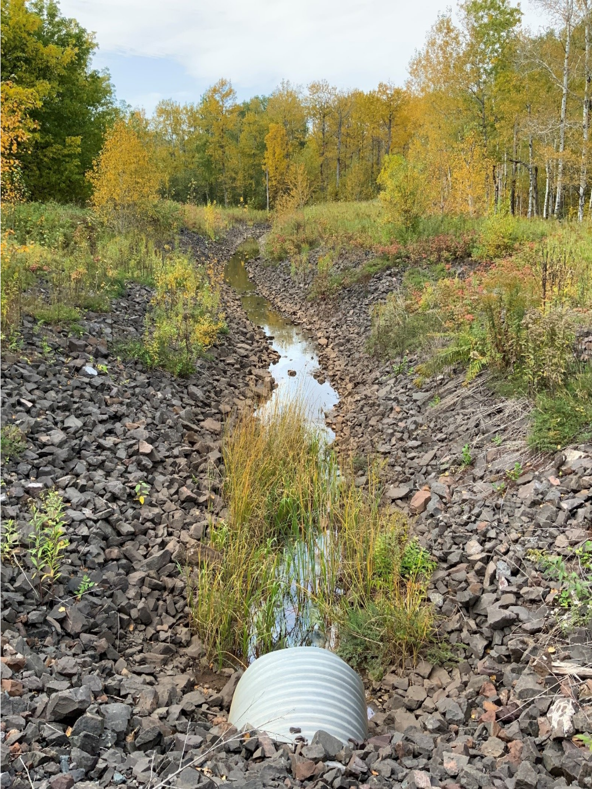
Outfall 001 Drainage Ditch Photo 3, looking West from center area:
