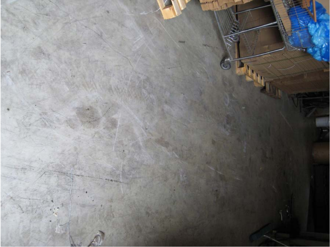
Floor sealant inside former Doberstein Lumber and Fence building Photograph taken 08/21/08
