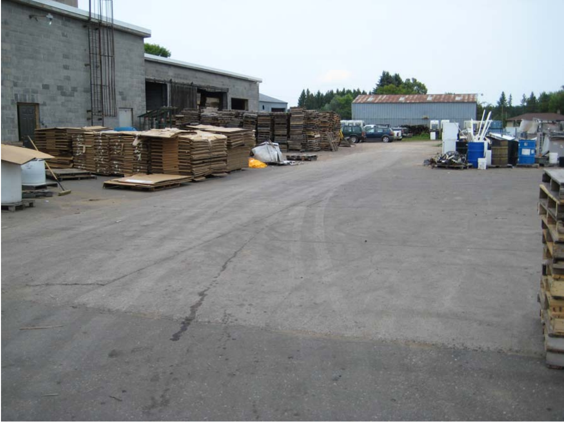
East side of former Doberstein Lumber and Fence building Looking north Photograph taken 08/21/08
