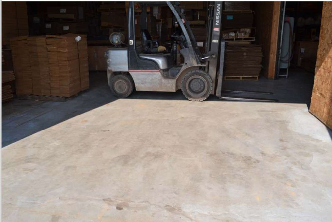
Title: Doberstein looking west into the building at floor sealent
