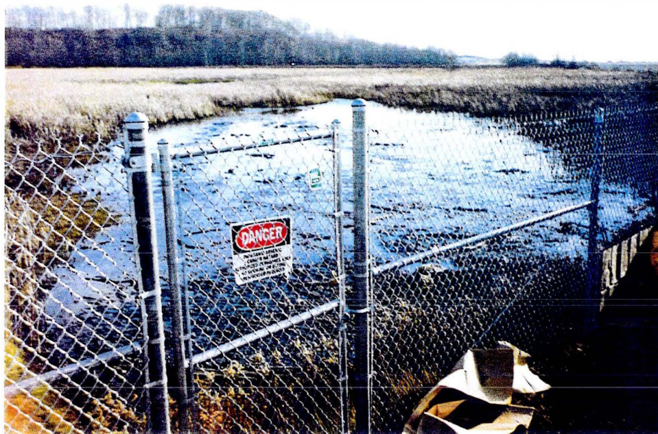
Photo 2: Security Fence and Hazard Warning Signs
