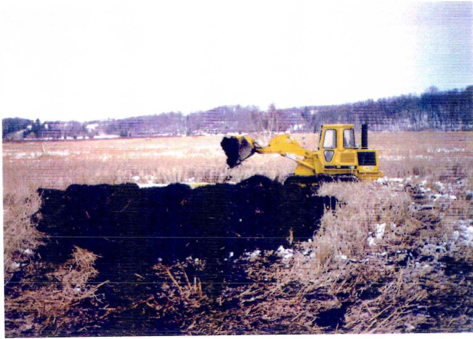
Photo 18: Woodchip placement in depressions.
