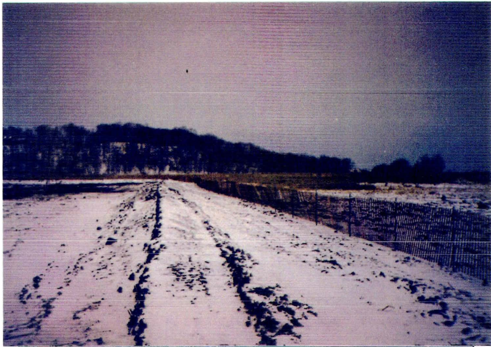
Photo 16: Woodchip placement over fill material.
