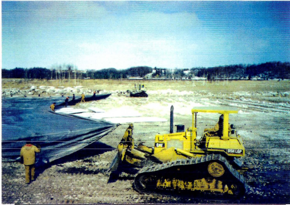
Photo 10: Pulling fabric over polystyrene blocks.
