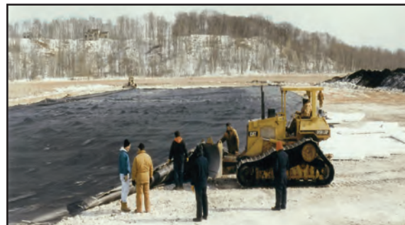
Crews install a cap over contamination at the site.
