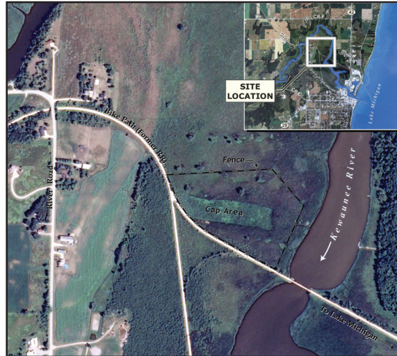
An aerial view of the site.
