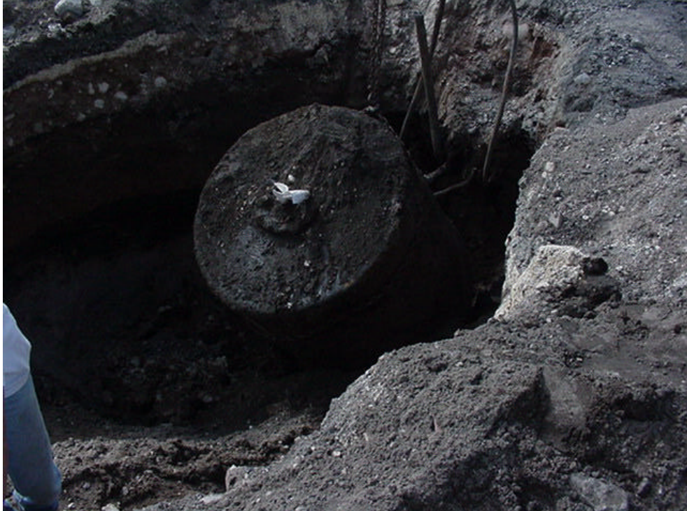
Photograph 3: Removal of UST #2.
