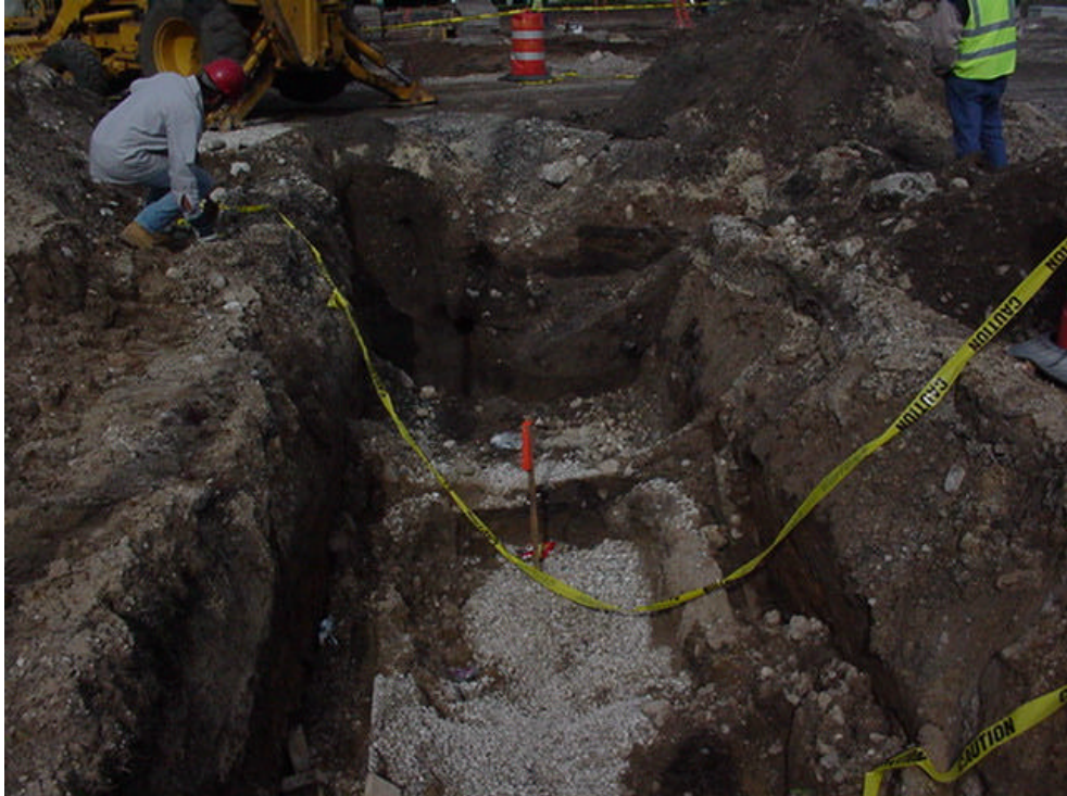
Photograph 1: UST #1 location related to the sewer construction trench.
