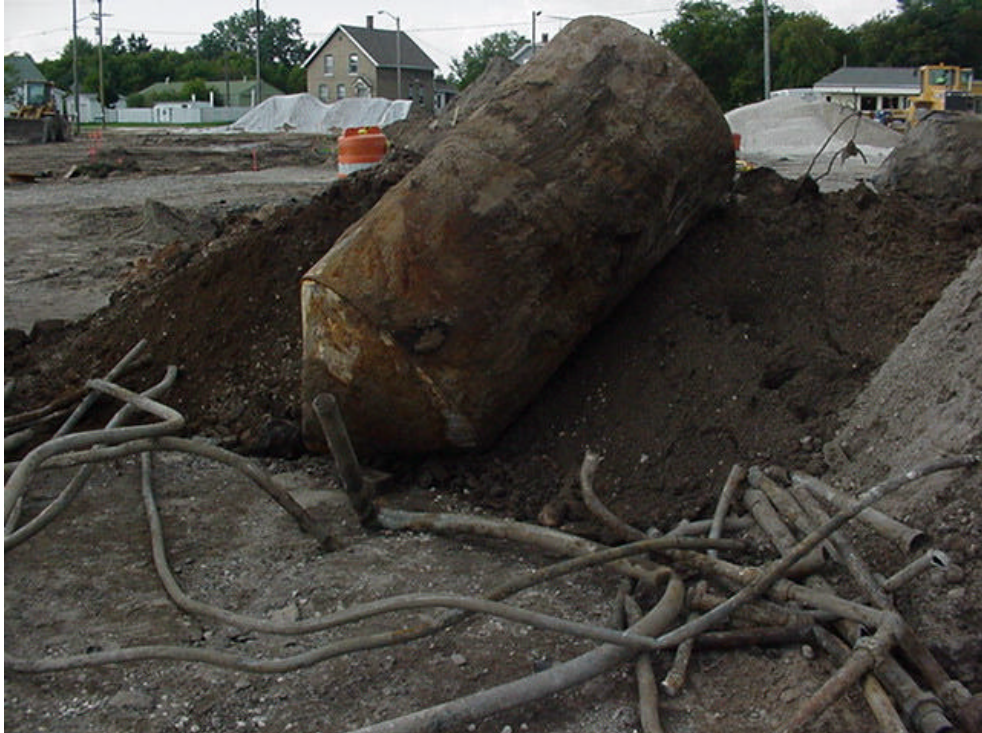
Photograph 5: UST #3 and associated piping after removal.
