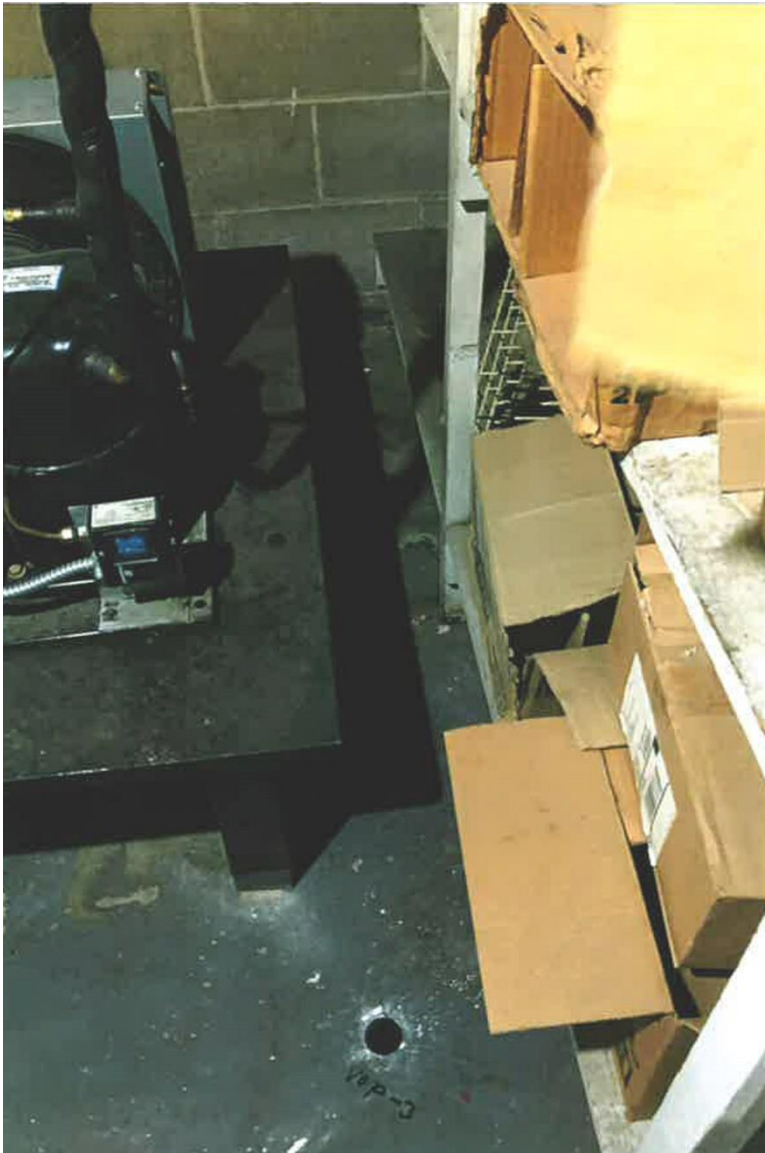
Photo 11: Sub-slab vacuum observation point VOP-3.
