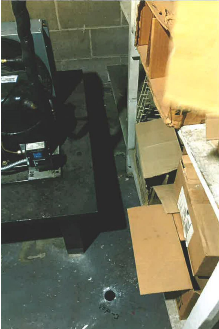
Photo 11: Sub-slab vacuum observation point VOP-3.
