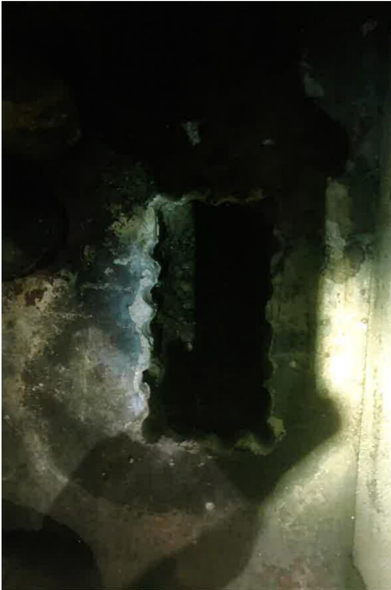
Photo 2: Excavation through floor slab at Pickup Point 2.
