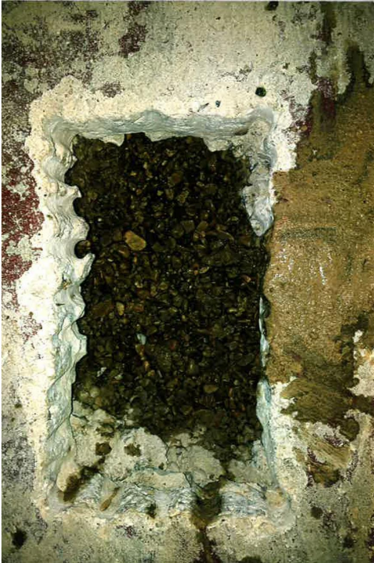
Photo 1: Excavation through floor slab at Pickup Point 1.
