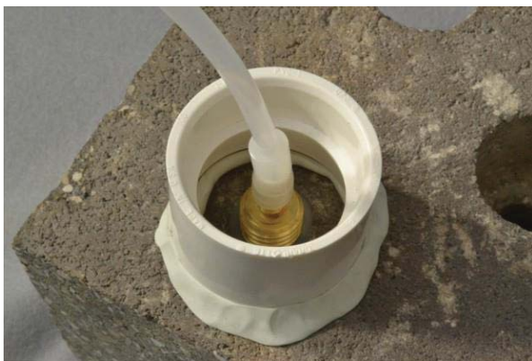
Figure 6. Water dam used for leak detection
