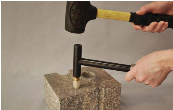
Figure 2. Installing the VAPOR PIN®
