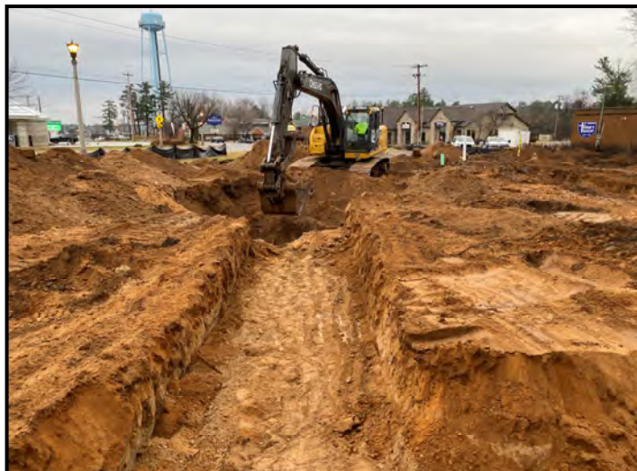
Footing excavation, view to north
