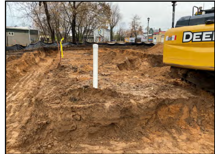
Water and sewer riser, footing excavation
