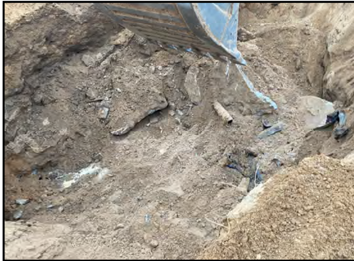
Former building foundation encountered during footing excavation
