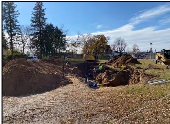
Laying sewer and water pipe
