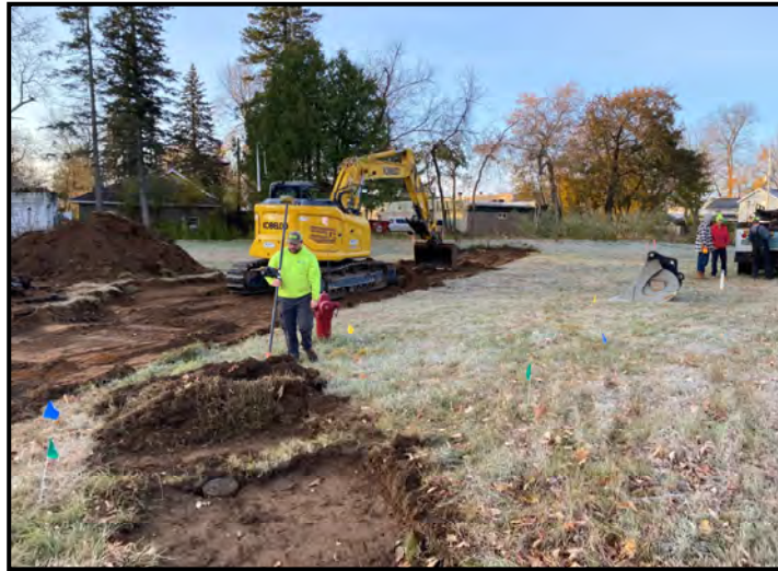
Stripping topsoil for water/sewer trench
