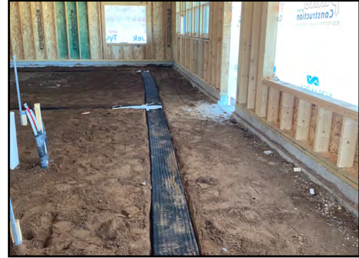
Gas Mat being installed
