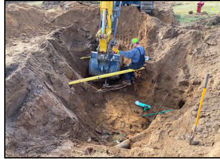
Trenching under gas line
