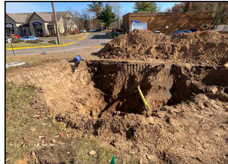
Connection at water main
