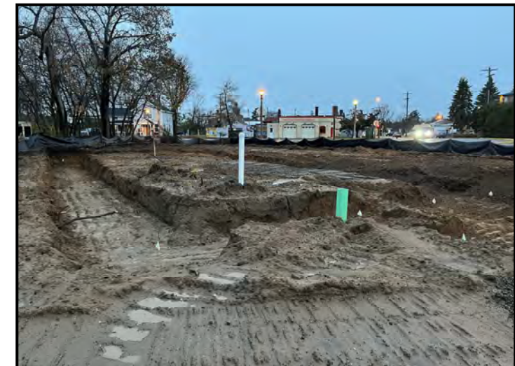
Completed footing excavation, sewer and water and cleanout risers
