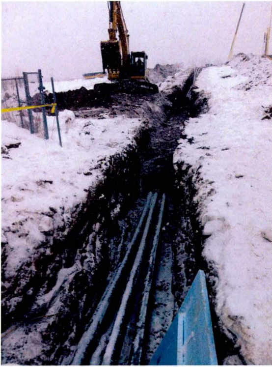
Conveyance pipe excavation will piping installed – looking west toward the CAMU
