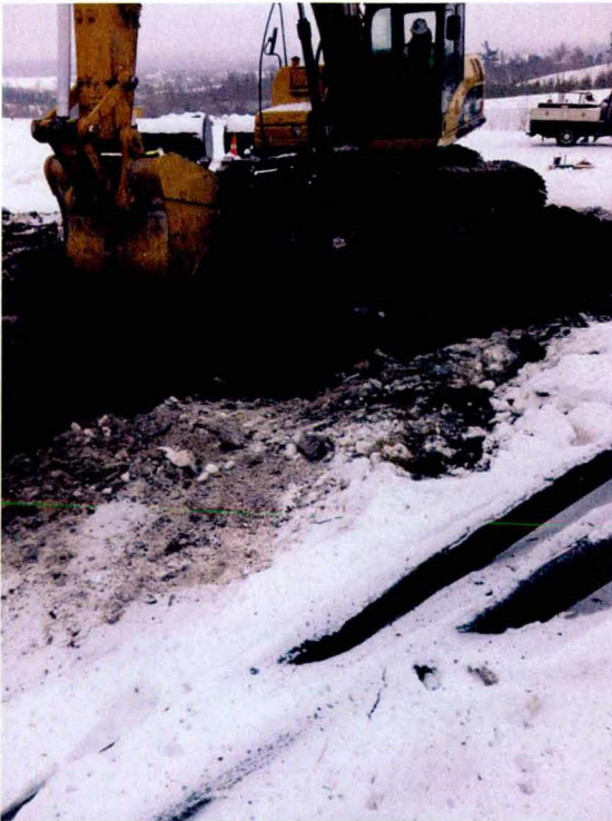
Excavation for the vault around EW-12 – looking east
