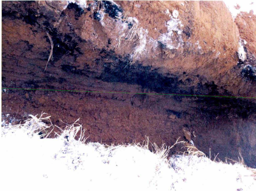
Conveyance pipe excavation
