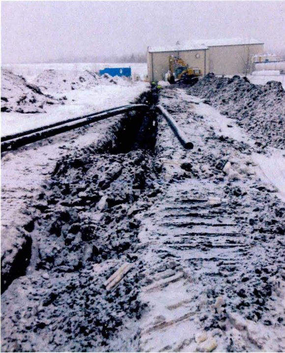
Conveyance Piping Installation looking east toward the Treatment Plant
