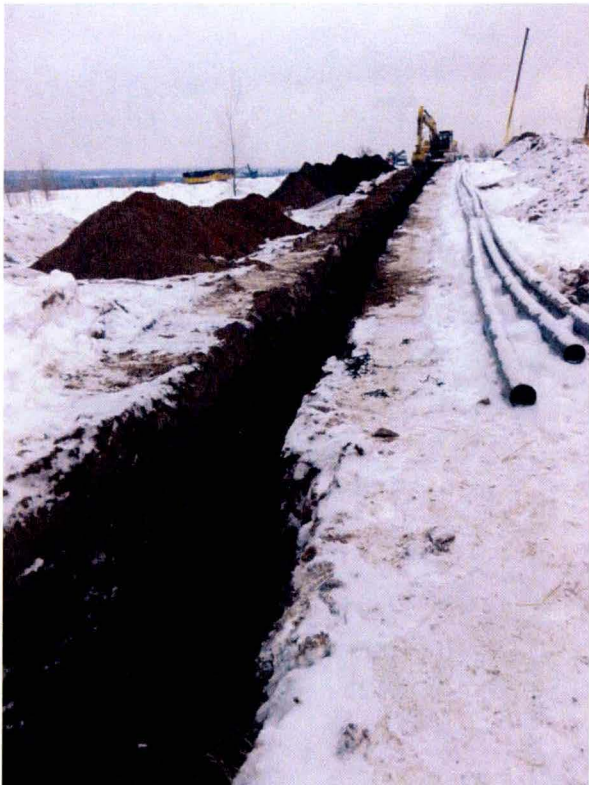
Conveyance Pipe excavation – looking west toward the CAMU
