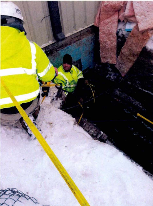
Coupling the HDPE piping at the conveyance piping penetration point
