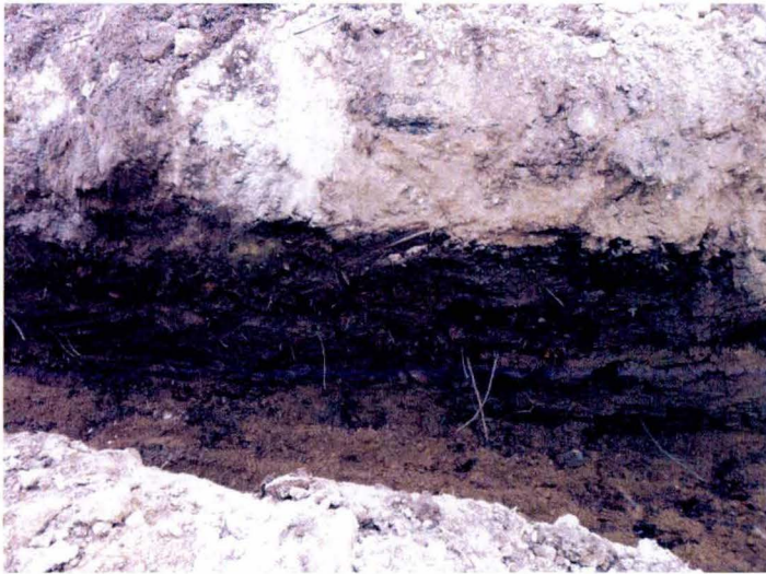
Conveyance piping excavation – soil layering
