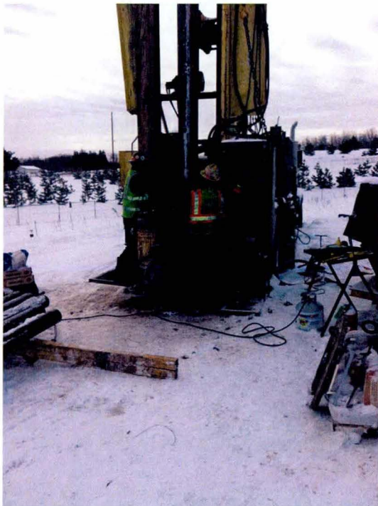
Barbary Rig Drilling at EW-13 – looking southwest
