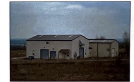
TREATMENT BUILDING AT PENTA WOOD PRODUCTS SITE
