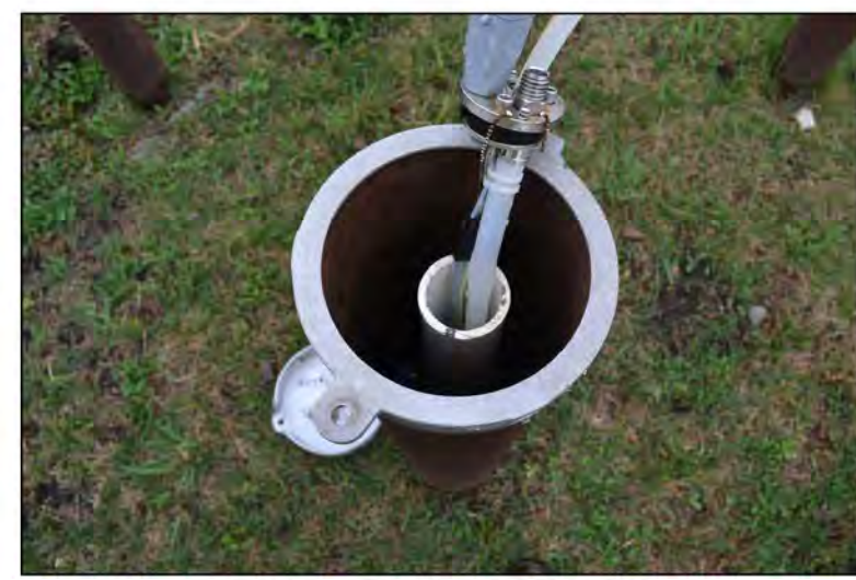
UNCONFINED MONITORING WELL
