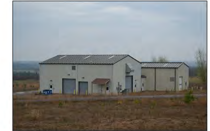
TREATMENT BUILDING AT PENTA WOOD PRODUCTS SITE
