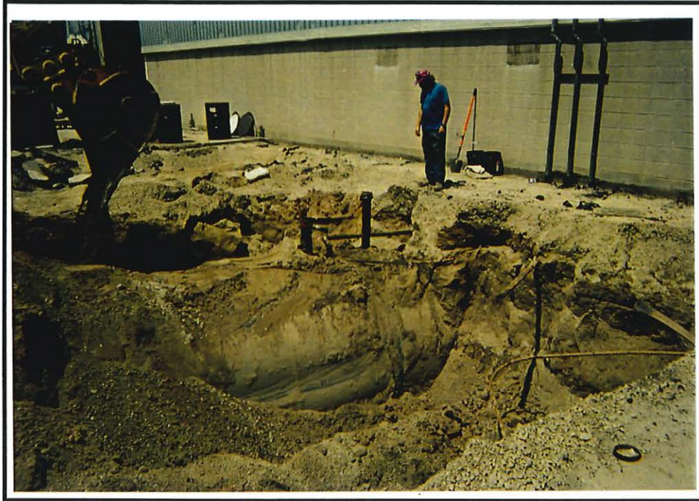
Removal of the Diesel UST.
