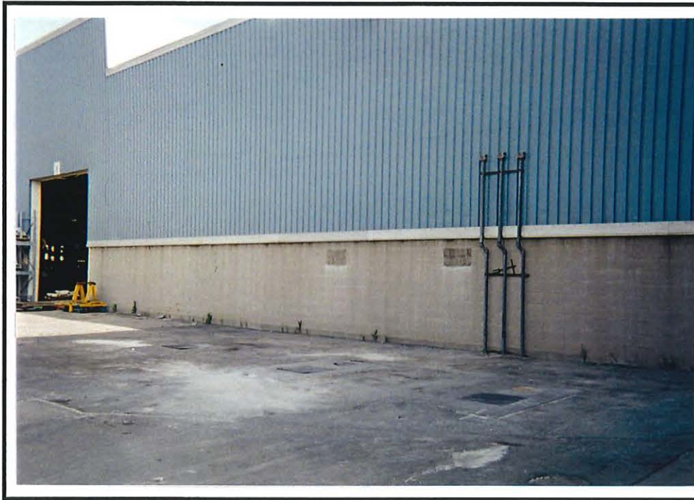
Site conditions before excavation.
