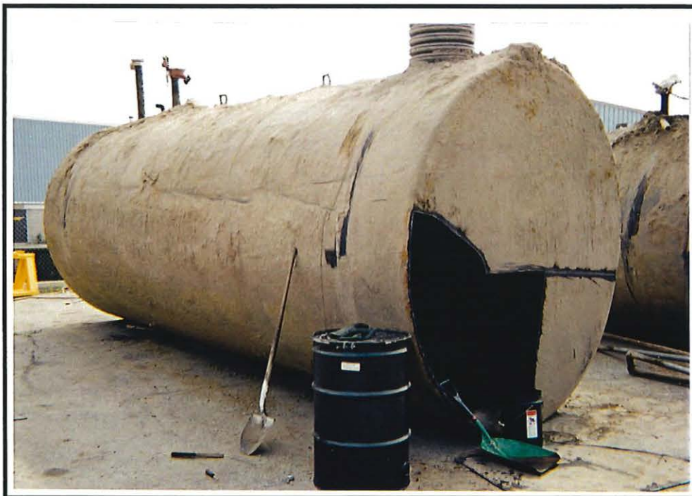
The Diesel UST after removal.
