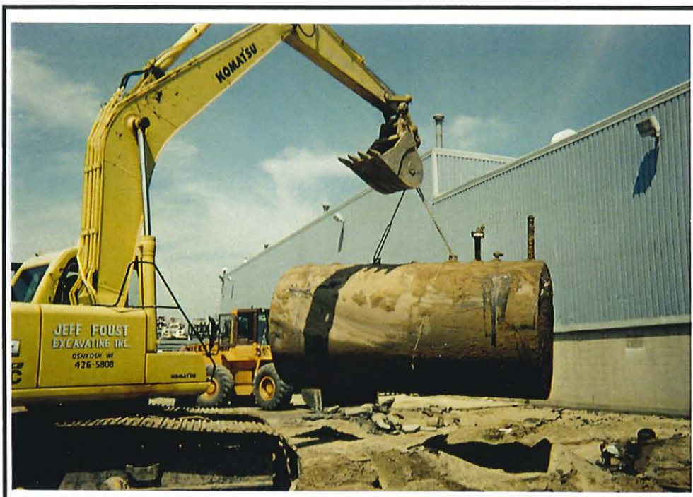
Removal of the Anti-Freeze UST.
