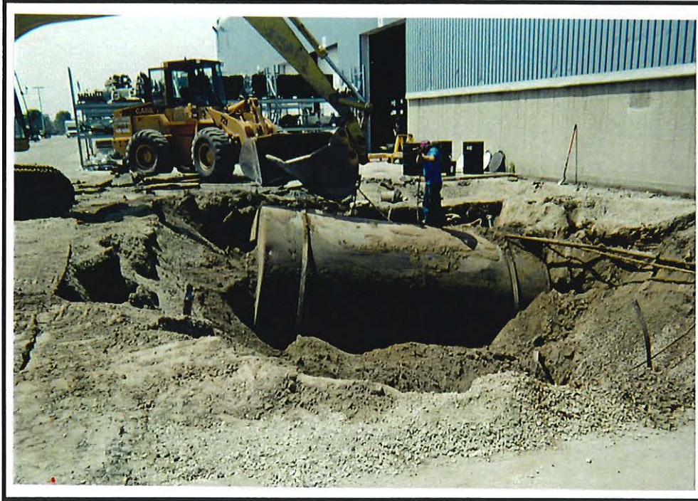
Removal of the Hydraulic Oil UST.
