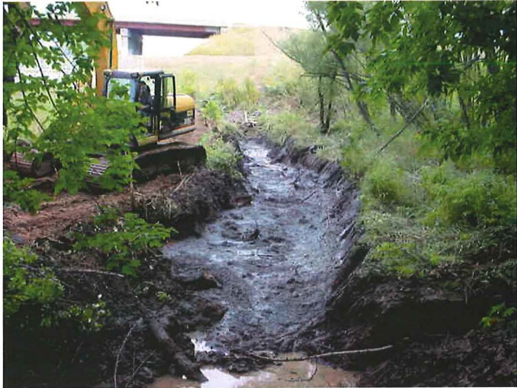
Photo 25 - Segment KIV, looking east
