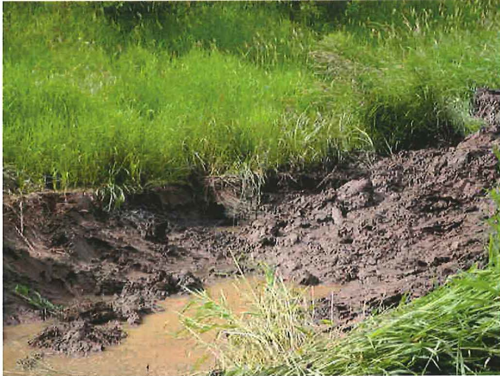
Photo 5 - Segment CVII Creek Channell – Excavation of Saturated Material
