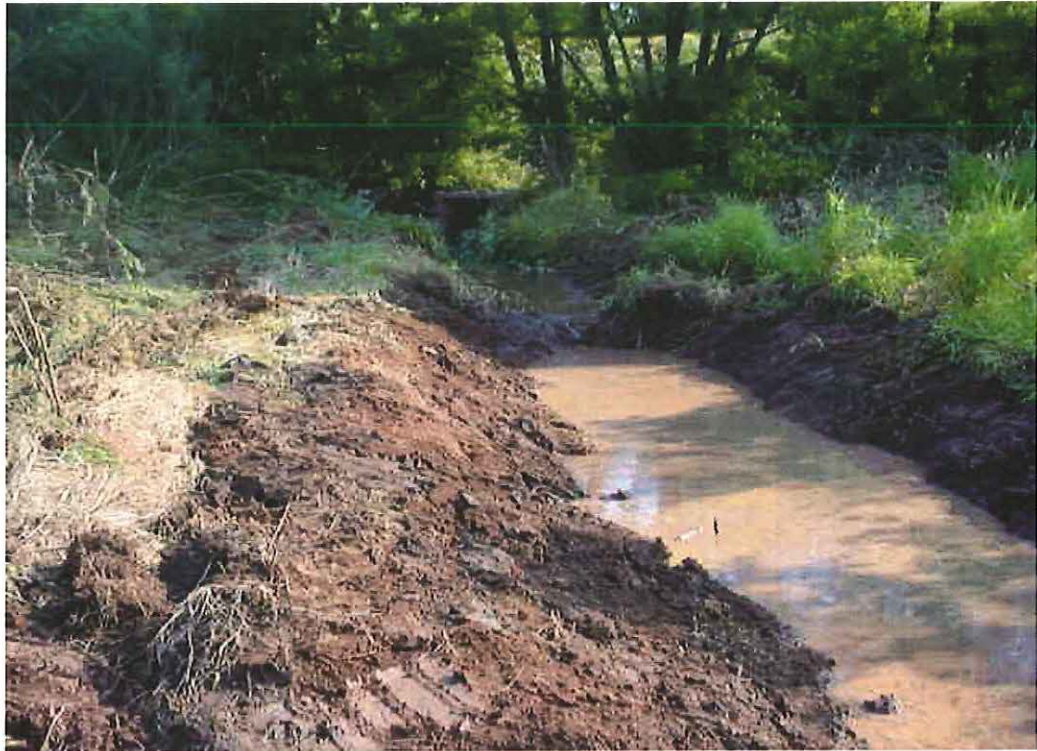
Photo 19 - Segment GIV, looking east
