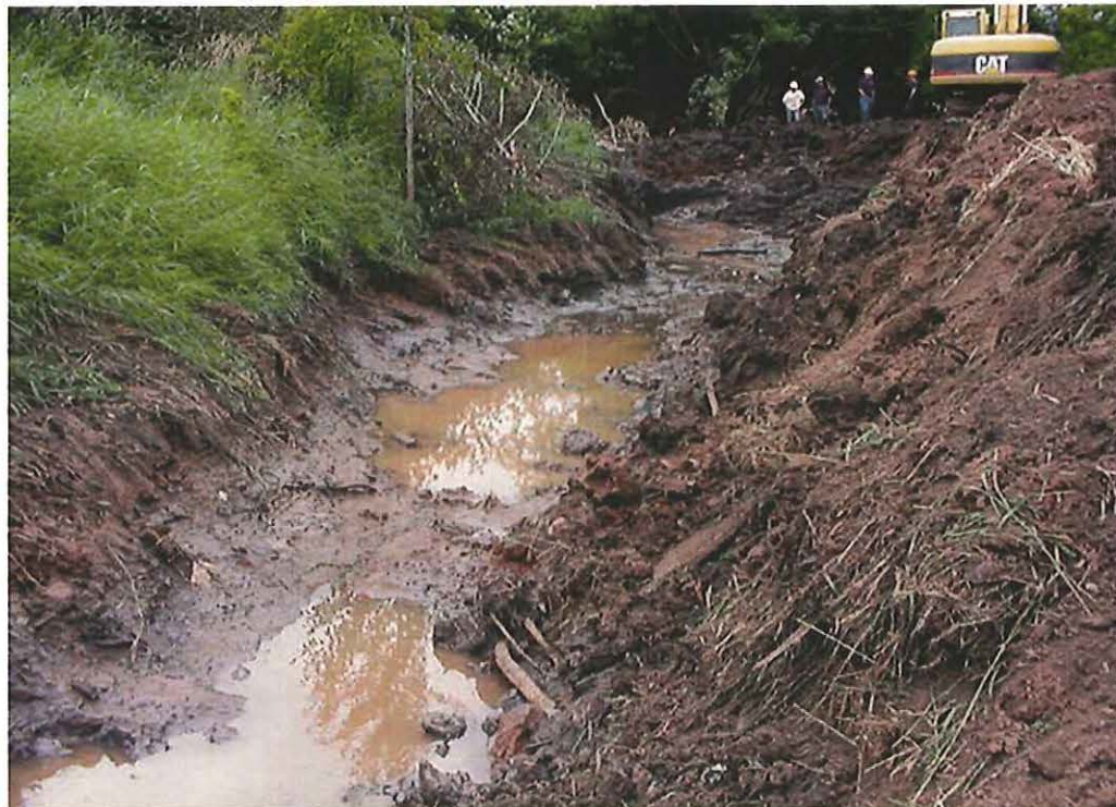
Photo 12 - Segment FVI, looking west
