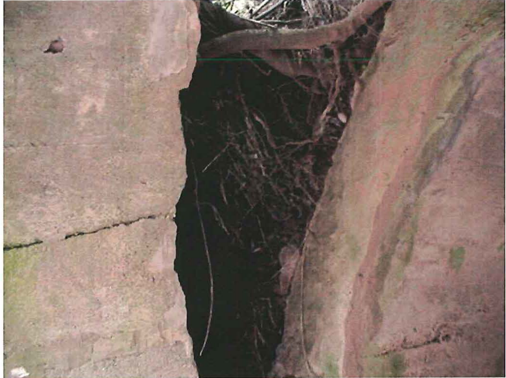
Photo 15 - Segment FVII Culvert
