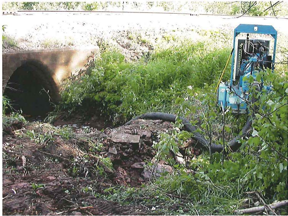
Photo 2 - Basin Bypass July 2003.
