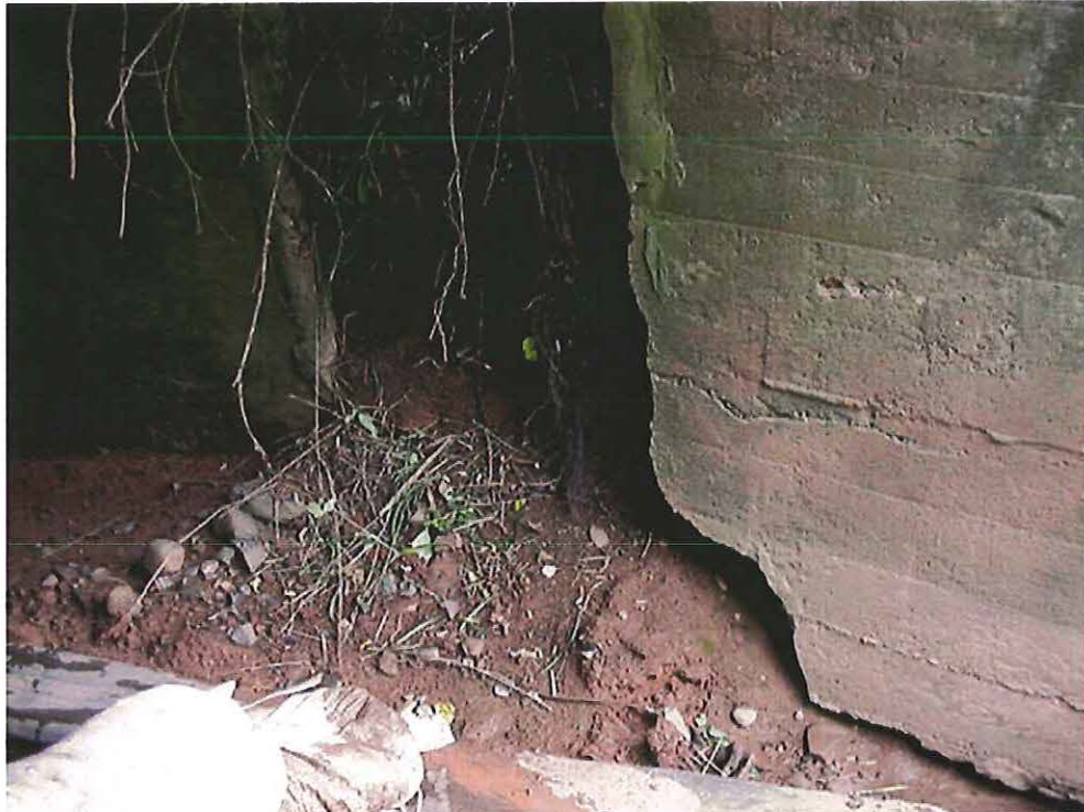
Photo 13 - Segment FVII Culvert
