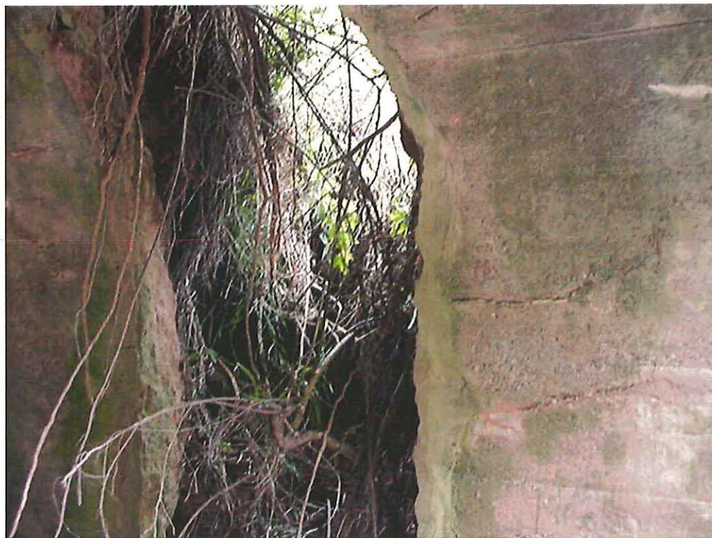
Photo 14 - Segment FVII Culvert
