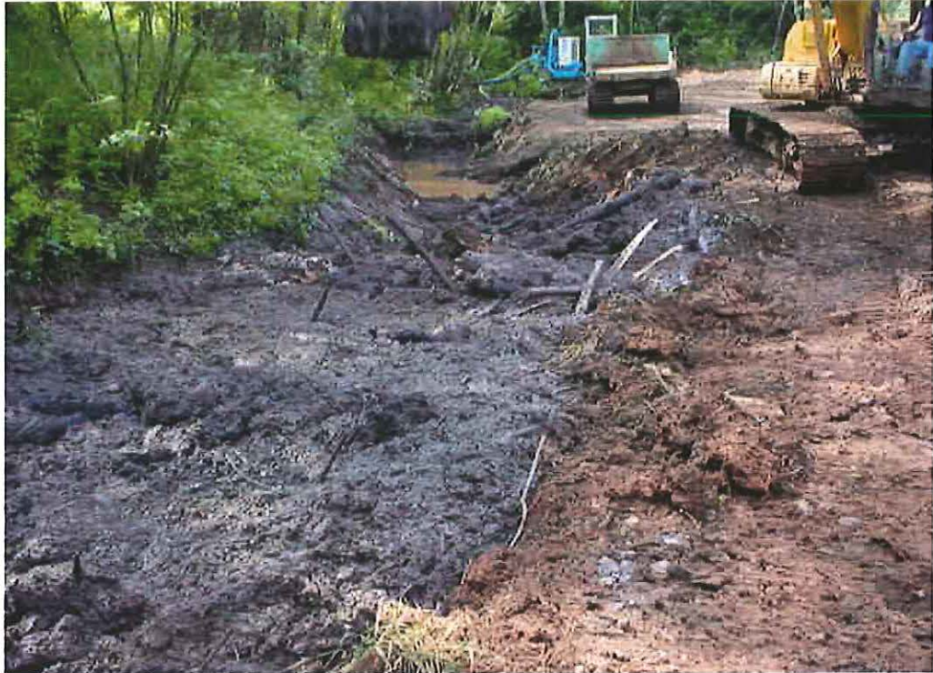
Photo 23 - Segment J, looking west
