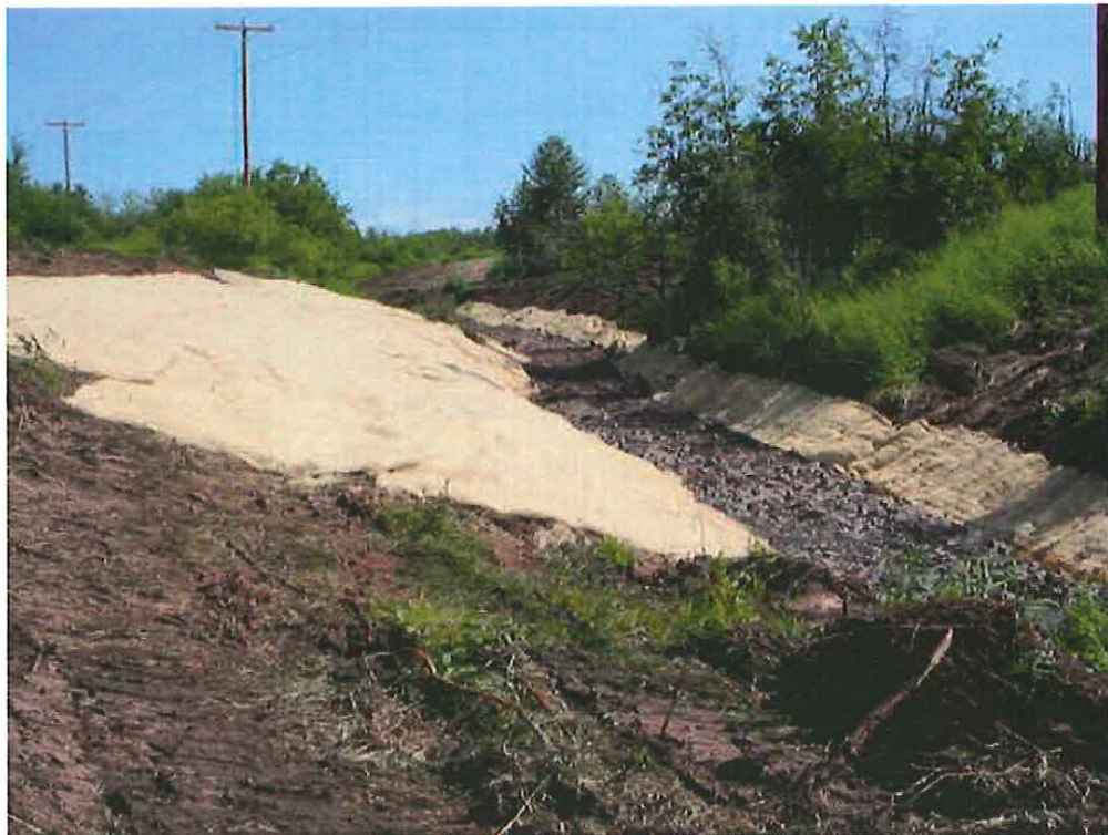
Photo 6 - Segment CV Restoration.
