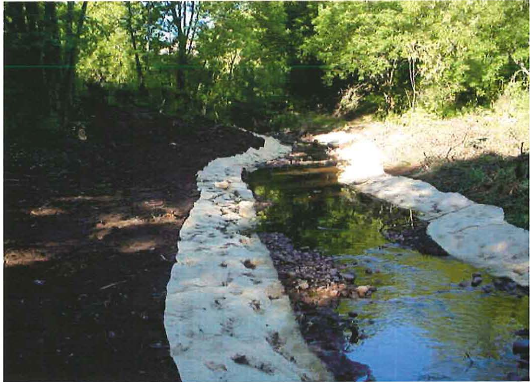
Photo 21 - Segment HIII, looking west
