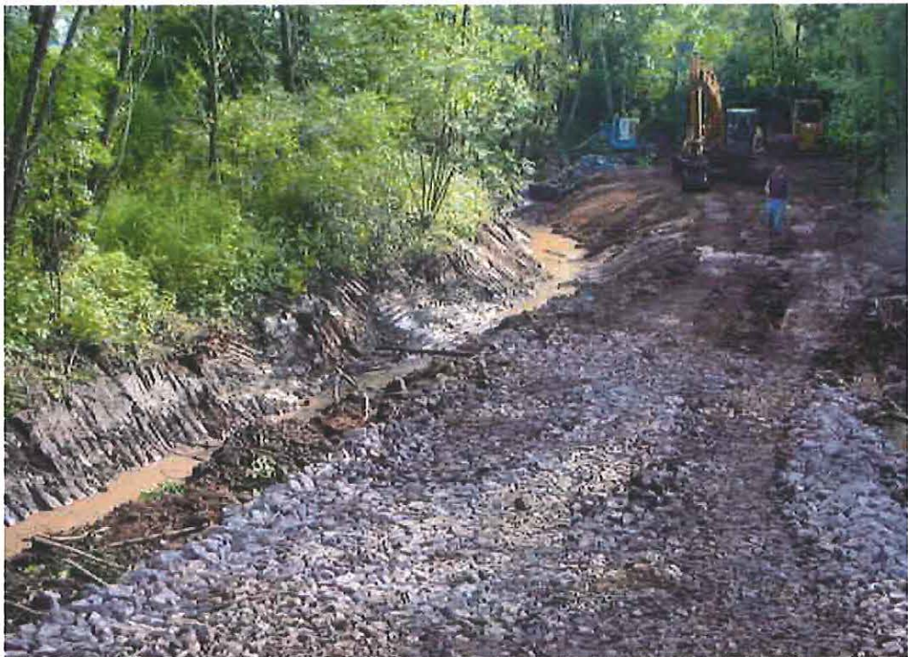
Photo 24 - Segment J, looking west
