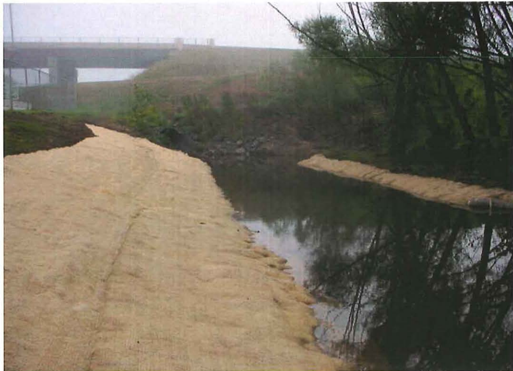
Photo 26 - Segment KIV, looking east
