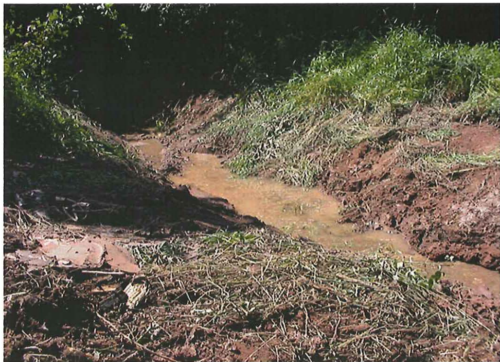
Photo 10 - Segment EI, looking west
