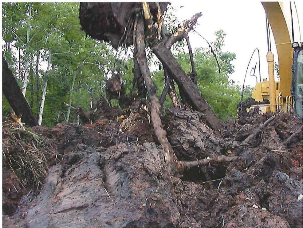
Photo 4 - Segment BIX Railroad Ties In Creek
