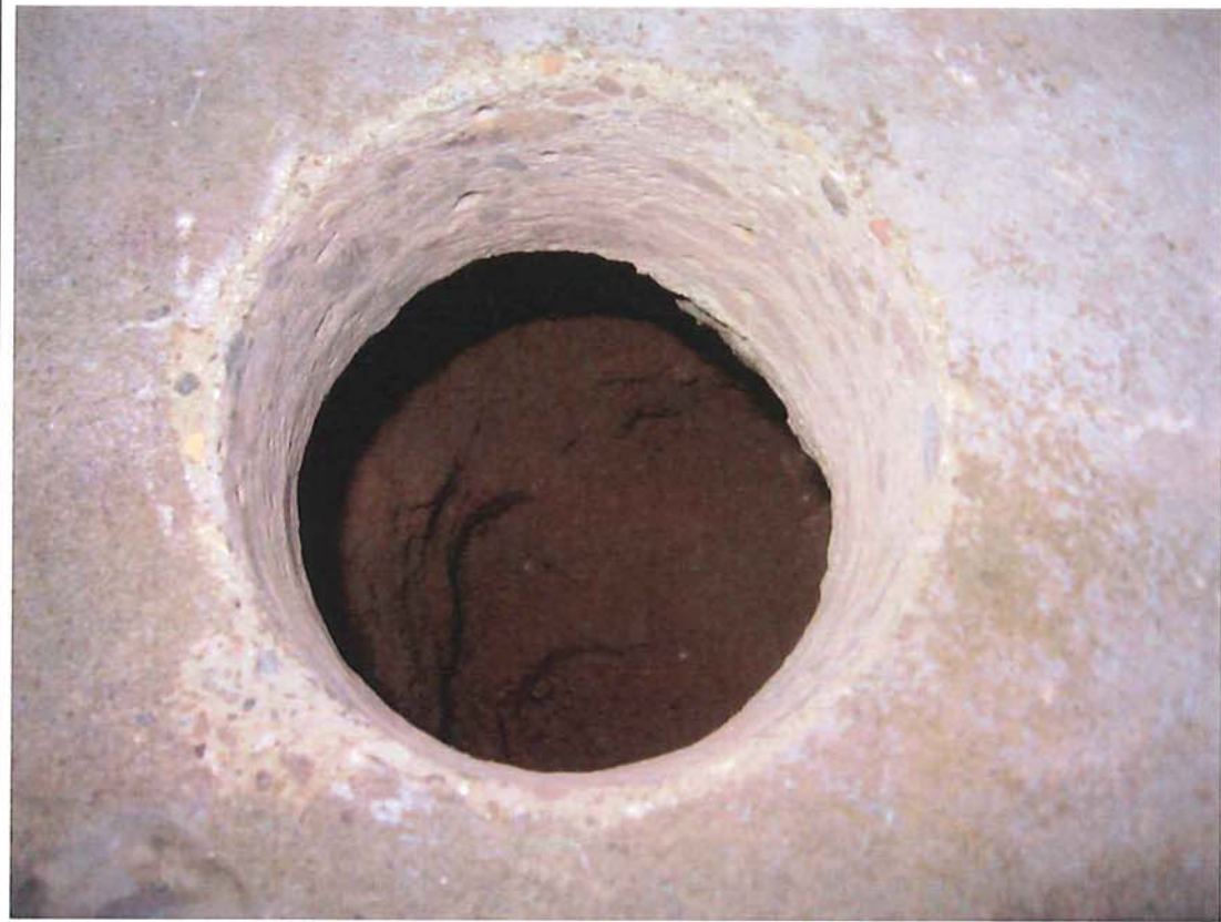
Photograph #: 1 Date: 9/25/2012 Direction: System #1 Subject: Cored hole to sub-slab material
