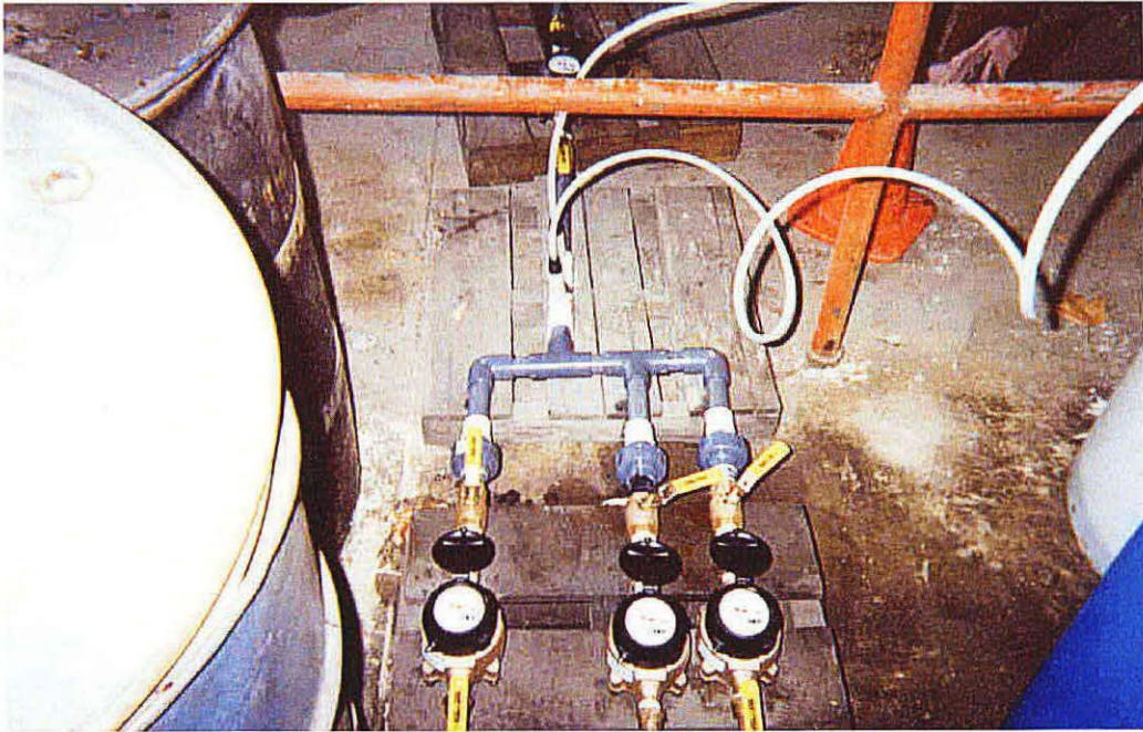
Photo No. 30 - Looking south, picture of the three flow meters that control the lactate injection flow rate to the three injection wells. Notice the variation in the valve opening. This variation was required in order to maintain similar flow rates to the three wells.
