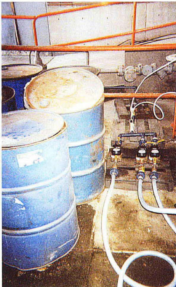
Photo No. 30 - Looking south, picture of the three flow meters that control the lactate injection flow rate to the three injection wells. Notice the variation in the valve opening. This variation was required in order to maintain similar flow rates to the three wells.
