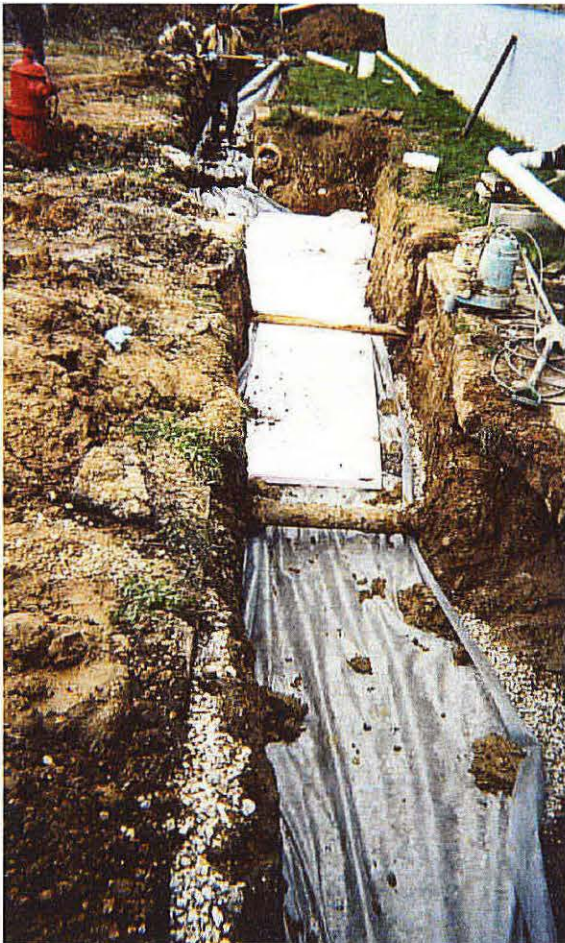
Photo No. 15 - Looking north, picture of the repaired sanitary sewer PVC pipe that had been damaged during the excavation of Trench 1.
