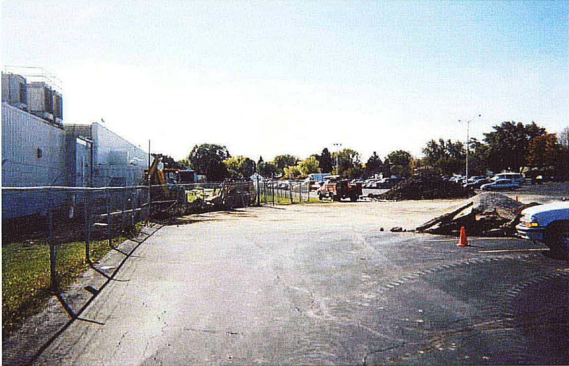
Photo No. 3 - Looking south, picture of the broken-up asphalt, removed for the installation of Trenches 3 and 4. The soil stockpile can be seen in the background.
