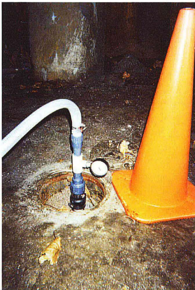
Photo No. 32 - Looking south, picture of the flexible hose that forms the connection between the chemical flow meters and the lactate injection wells. Orange cones are provided for safety.
