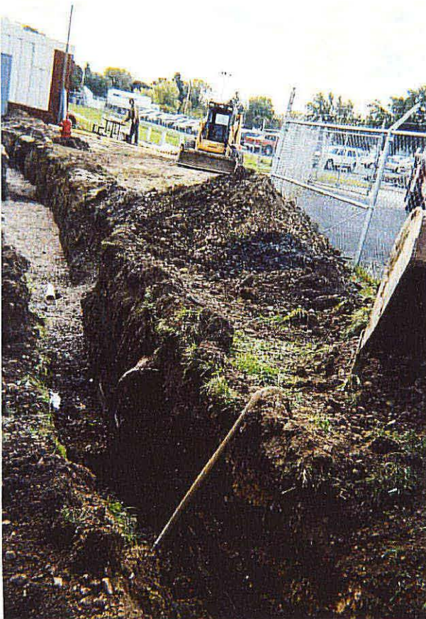
Photo No. 3 - Looking south, picture of the broken-up asphalt, removed for the installation of Trenches 3 and 4. The soil stockpile can be seen in the background.
