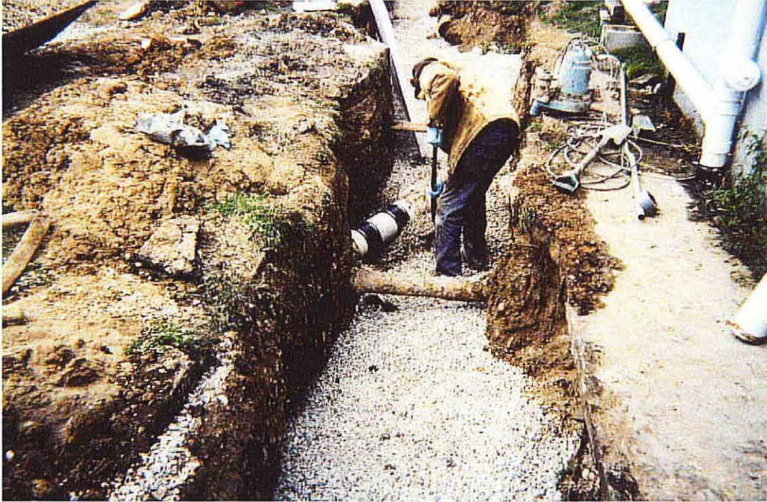
Photo No. 15 - Looking north, picture of the repaired sanitary sewer PVC pipe that had been damaged during the excavation of Trench 1.
