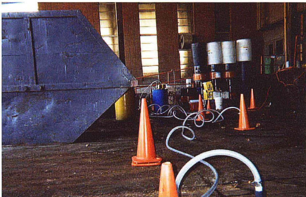
Photo No. 32 - Looking south, picture of the flexible hose that forms the connection between the chemical flow meters and the lactate injection wells. Orange cones are provided for safety.
