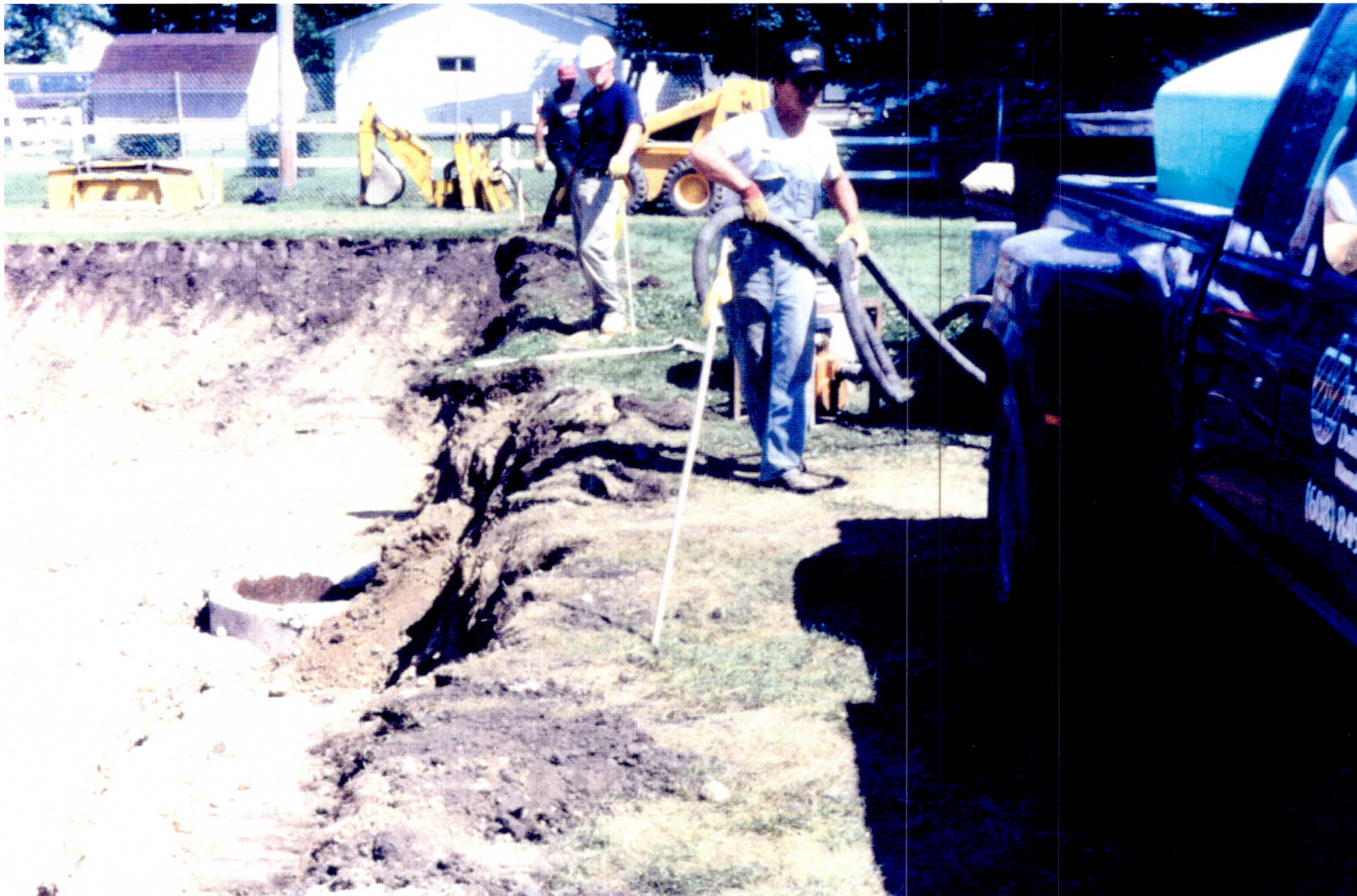
PHOTO NO. 2: ABANDONMENT OF WELL W-37 - BACKFILLING WITH BENTONITE SLURRY
