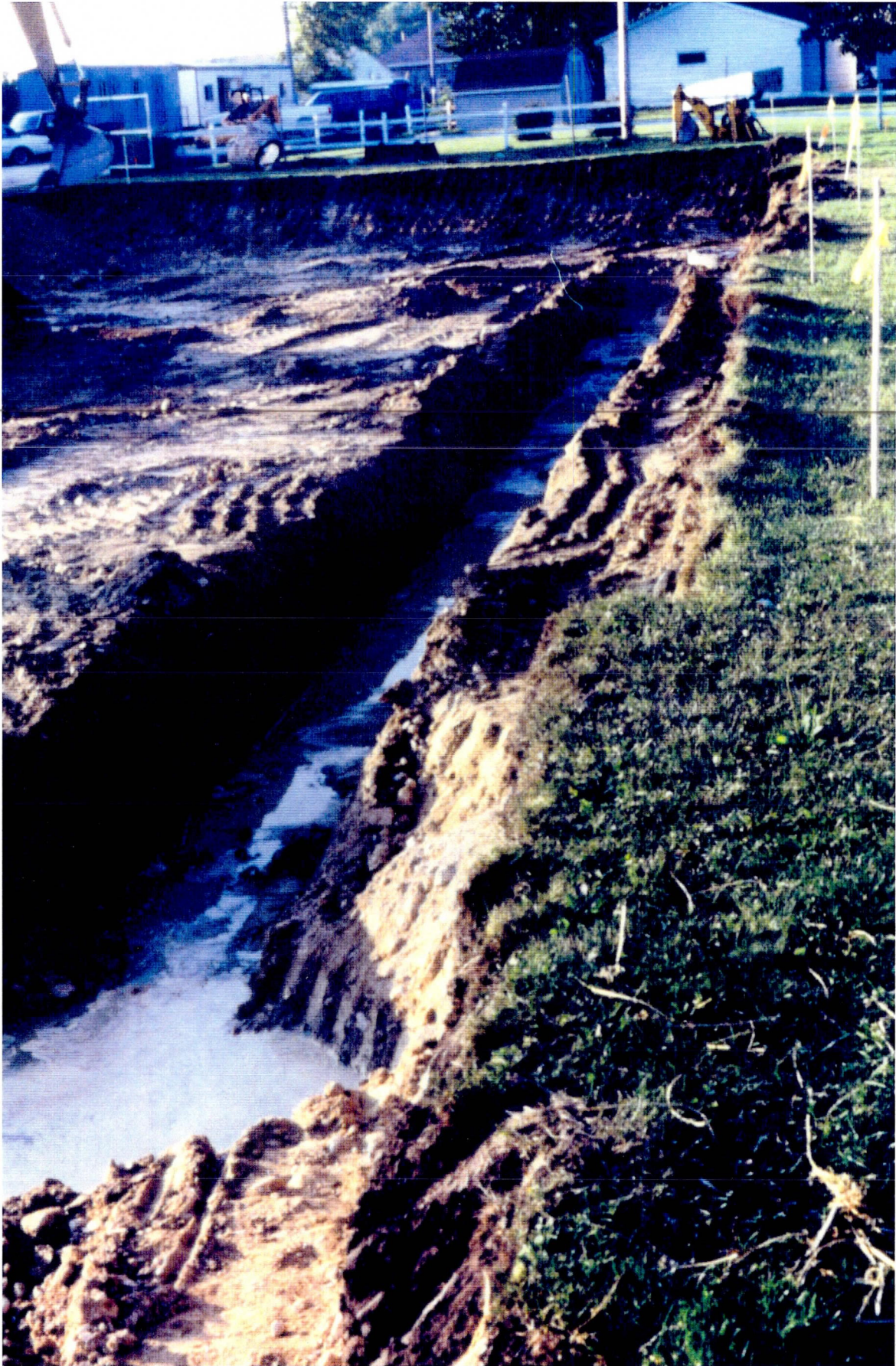
PHOTO NO. 3: RANNEY COLLECTOR TRENCH CONSTRUCTION AT W-37 LOOKING NORTH
