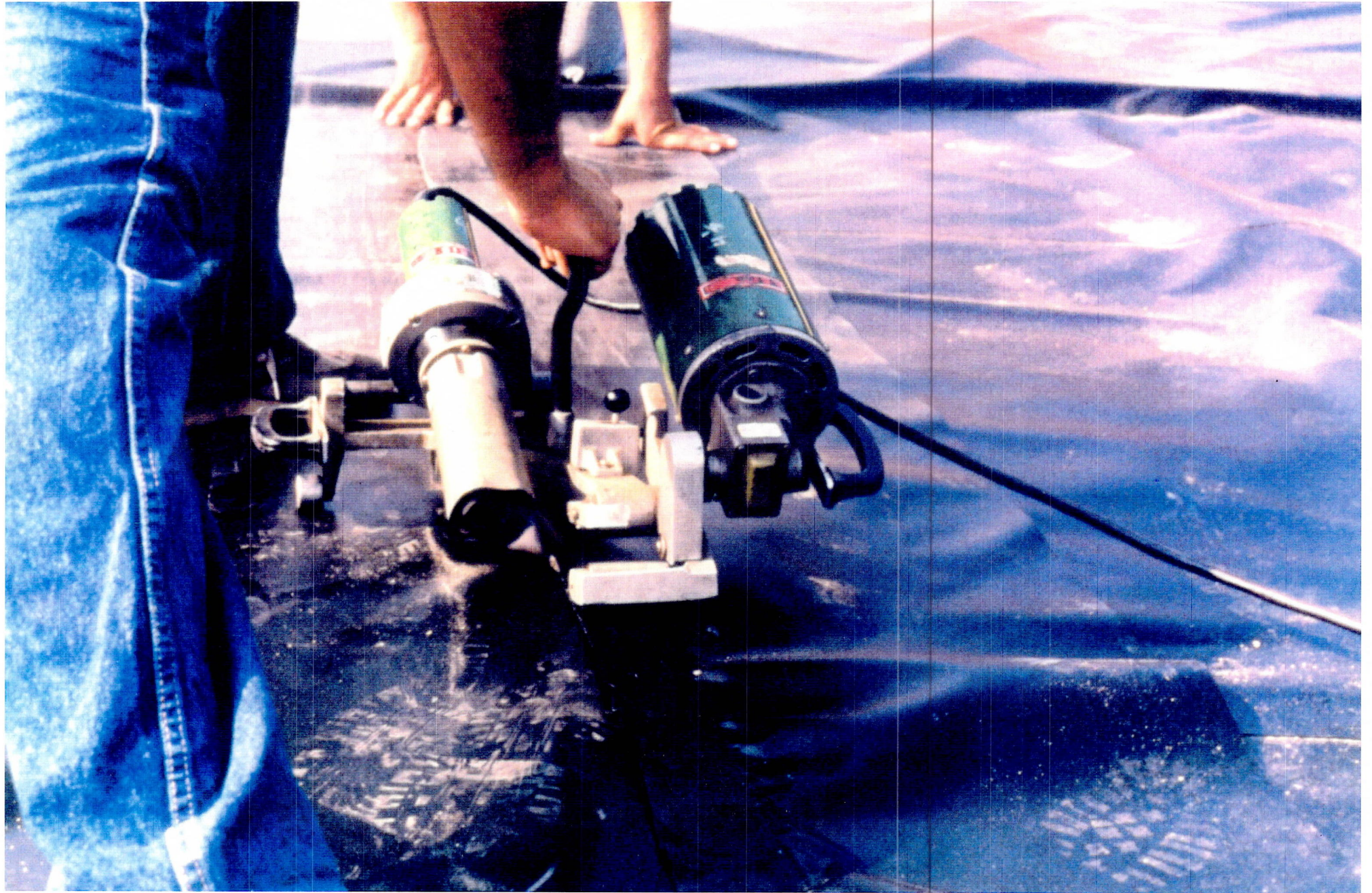
PHOTO NO. 5: GEOMEMBRANE LINER CONSTRUCTION - IN-FIELD SEAMING OF PANELS
