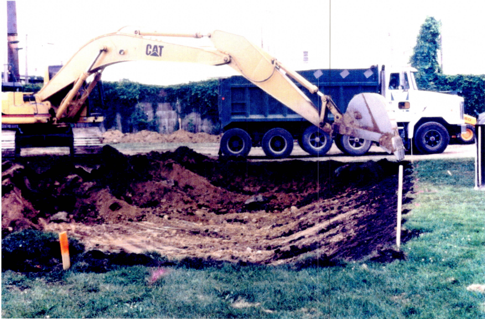
PHOTO NO. 1: TYPICAL EXCAVATION ACTIVITIES
