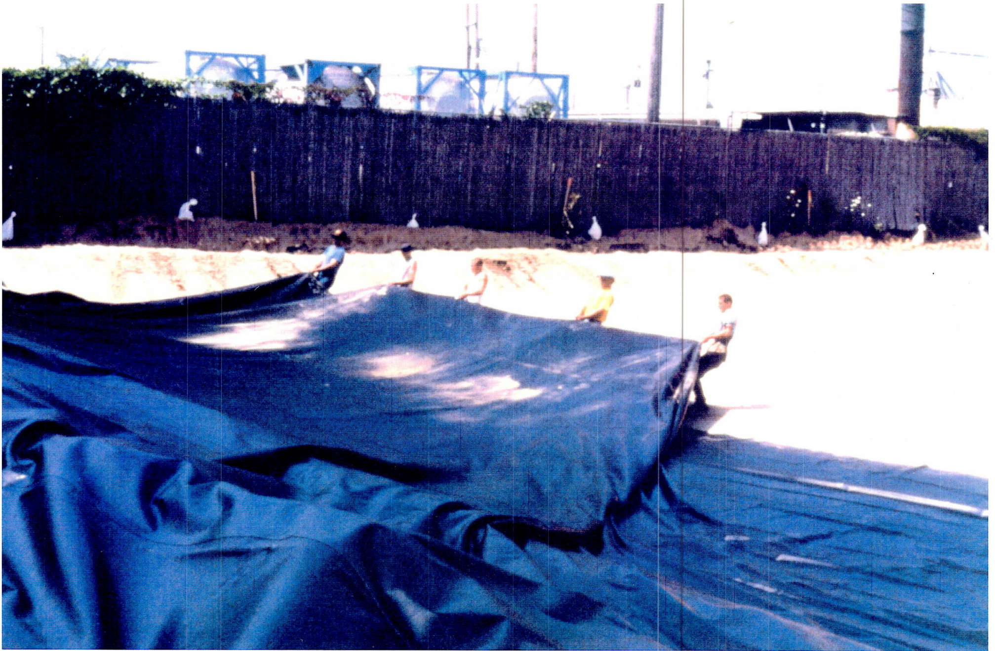
PHOTO NO. 4: GEOMEMBRANE LINER CONSTRUCTION - PANEL DEPLOYMENT
