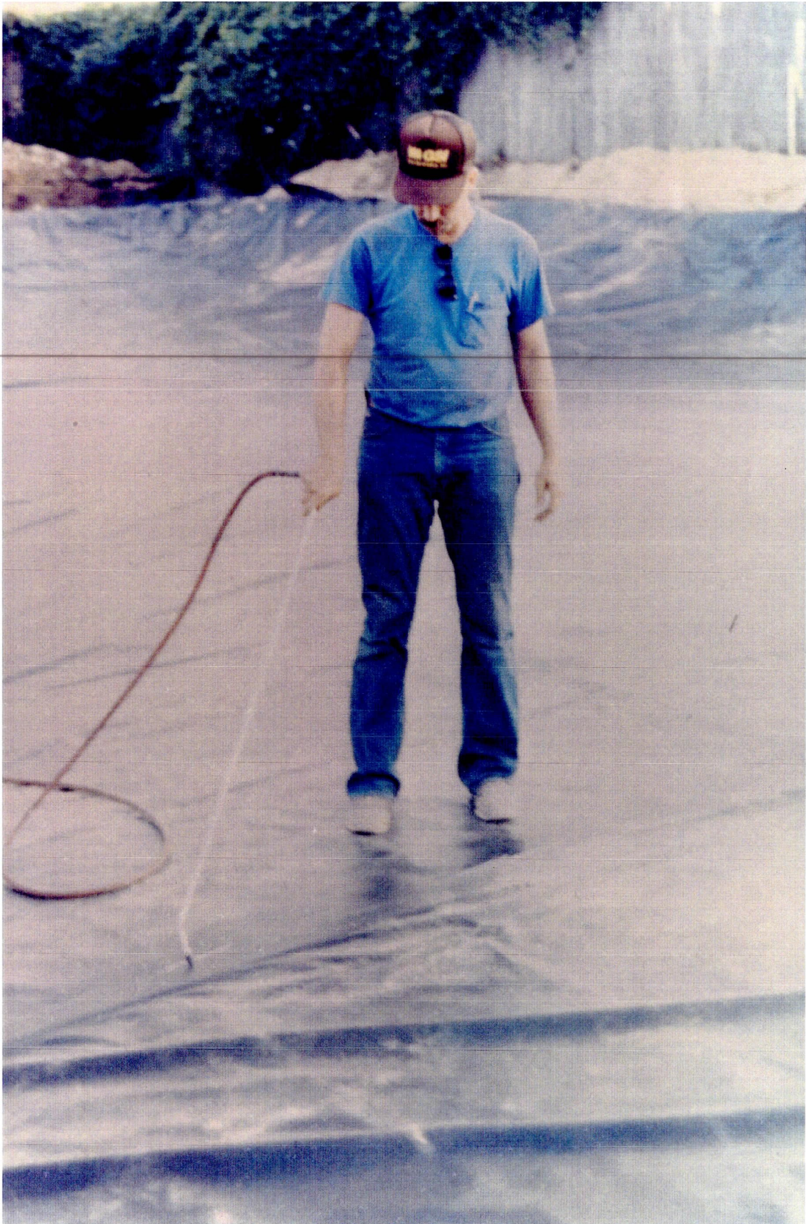
PHOTO NO. 6: GEOMEMBRANE LINER CONSTRUCTION - IN-FIELD SEAM TESTING
