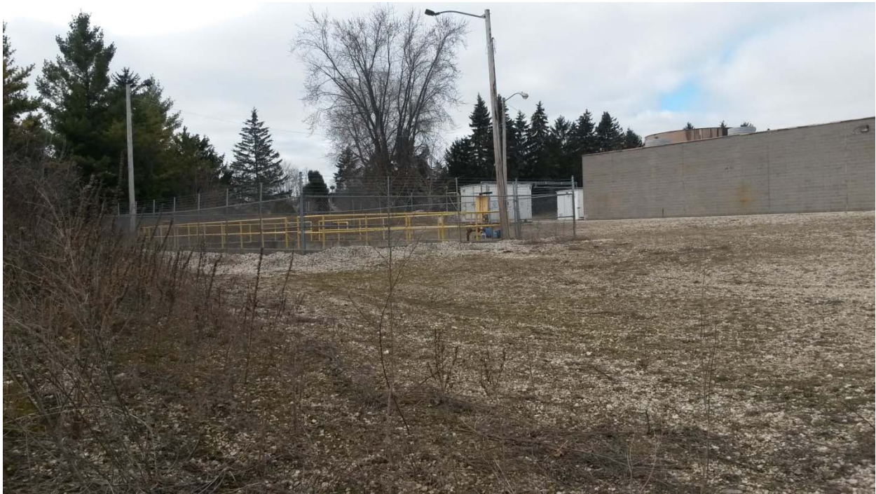
Photo 17. The pre-treatment pond.
