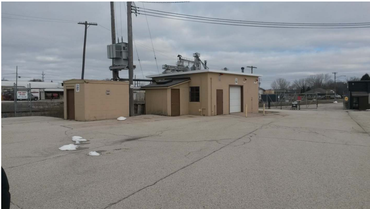
Photo 2. The building housing the deep extraction well and telemetry.
