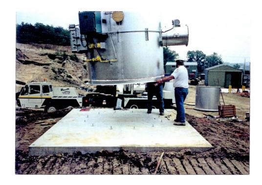
Photograph No. 10: Installing ground flare on slab. (Looking east) [mad-602-43g]
