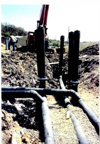
Photograph No. 8: Backfilling driplegs DL3 and DL4. (Looking east)
