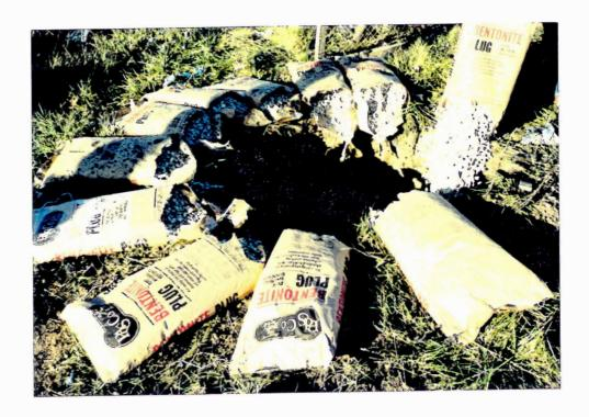
Photograph No. 3: Placing 1 ft bentonite seal at bottom of borehole.
