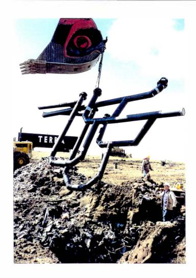
Photograph No. 7: Installing driplegs DL3 and DL4.
