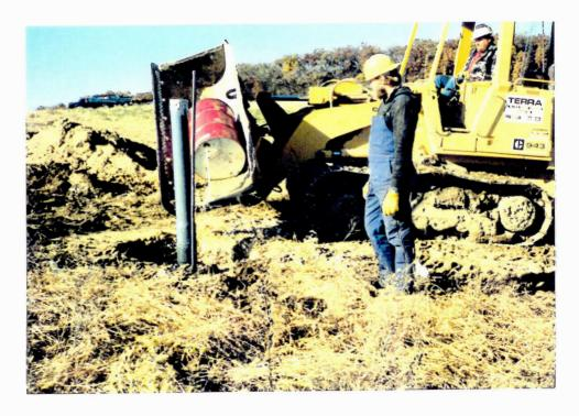
Photograph No. 4: Hydrating well seals with water.
