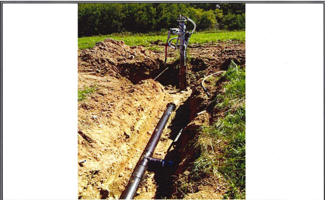
PHOTO: DATE: SUBJECT: 2 9/3/2014 GW-5 During Construction (Looking South)
