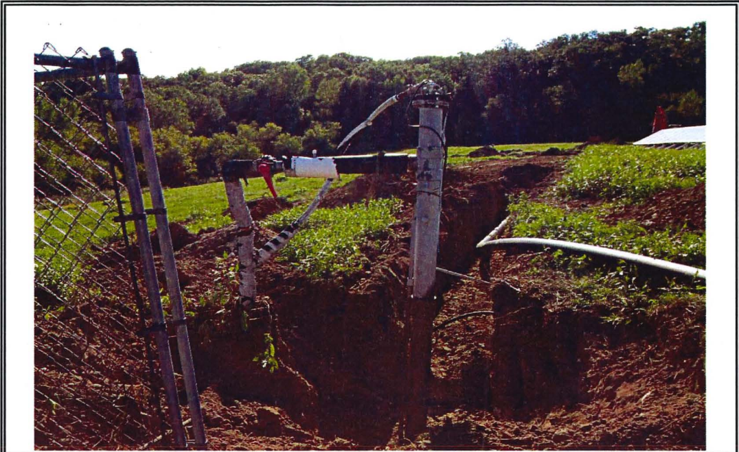
PHOTO: DATE: SUBJECT: 1 9/3/2014 GW-4 During Construction (Looking Northwest)
