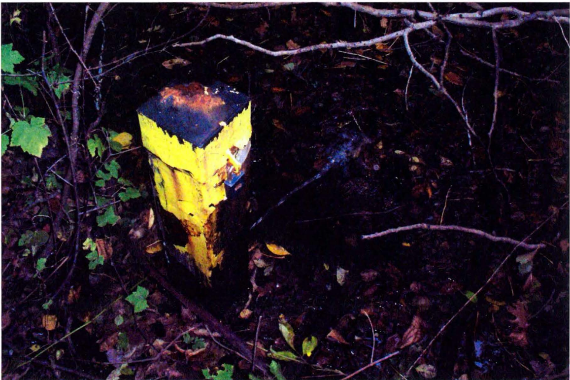
OW-4, View showing water seepage.
