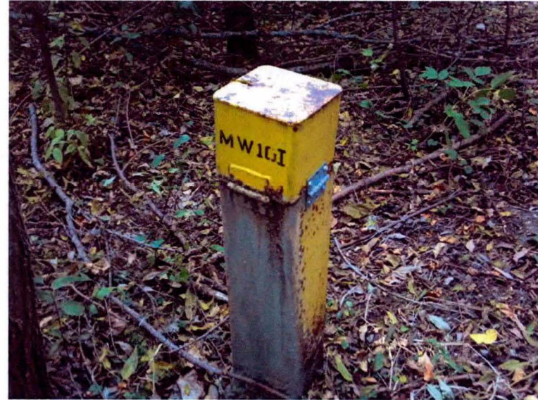
2012-09-008: MW101 – New Hinge Installed Date: 01-Oct-2012 Time: 8:06 AM Weather: Cloudy, 50 Degrees F.
