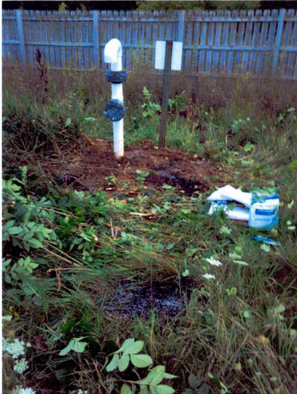
2012-09-003: GV-11 - Woody Root Mass Removed. Animal Burrow Plugged. Date: 26-Aug-2012 Time: 6:42 PM Weather: P-Cloudy, 75 Degrees F.
