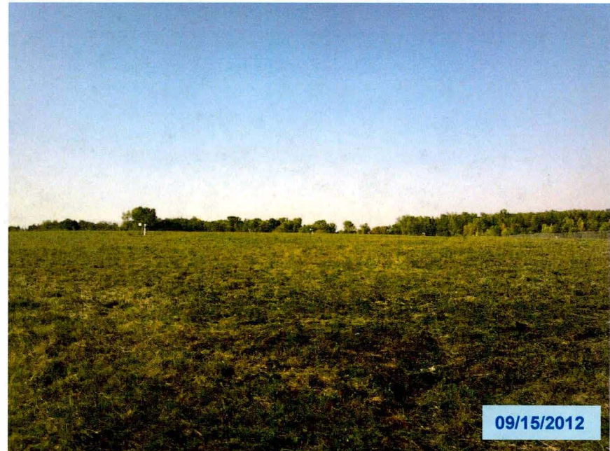
Landfill Cap – After Mowing
