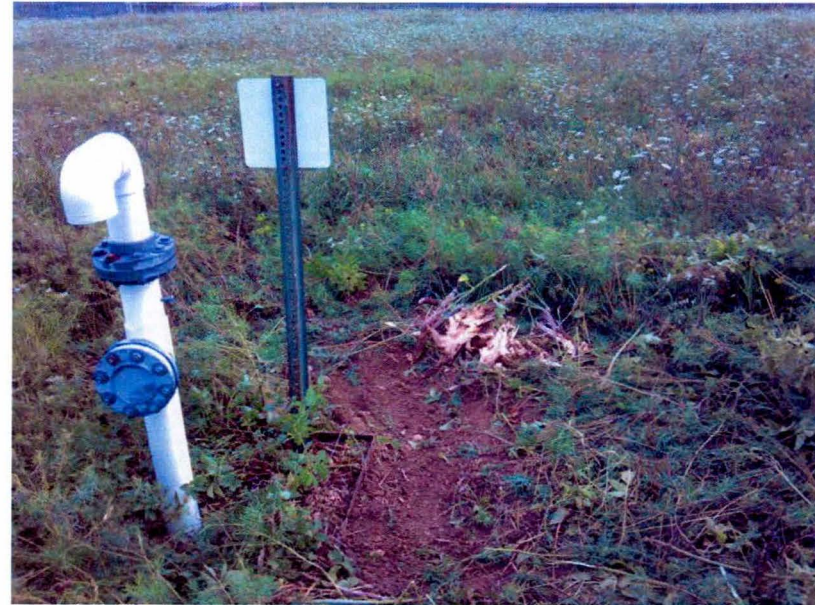
2012-09-002: GV-10 - Woody Root Mass Removed. Animal Burrow Plugged. Date: 26-Aug-2012 Time: 5:27 PM Weather: P-Cloudy, 80 Degrees F.
