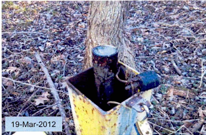
2011-10-013 : MW-10I protective casing hinge is broken, lock required replacement, and well needs a new expandable top
