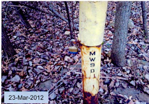
2011-10-011 : MW-9D – Lock was damaged and required replacement.
