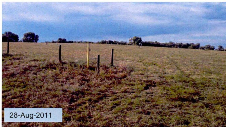
2011-10-027 : Finished conditions of the landfill cap following mowing event. MW-2 well nest is visible.
