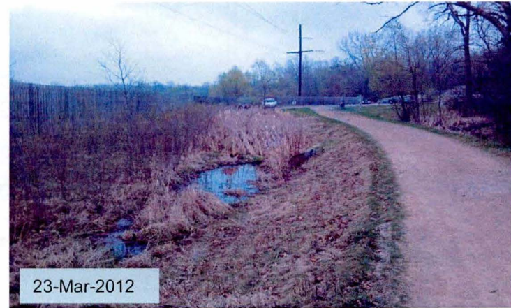
2011-10-030 : Cattails and woody vegetation in the south drainage feature.
