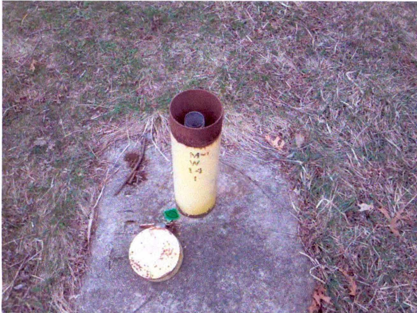
2012-10-015: MW14I – Well casing too high to allow installation of expandable cap Date: 23-Mar-2012 (Historical photo) Time: 2:51 PM Weather: Sunny, 35 Degrees F.
