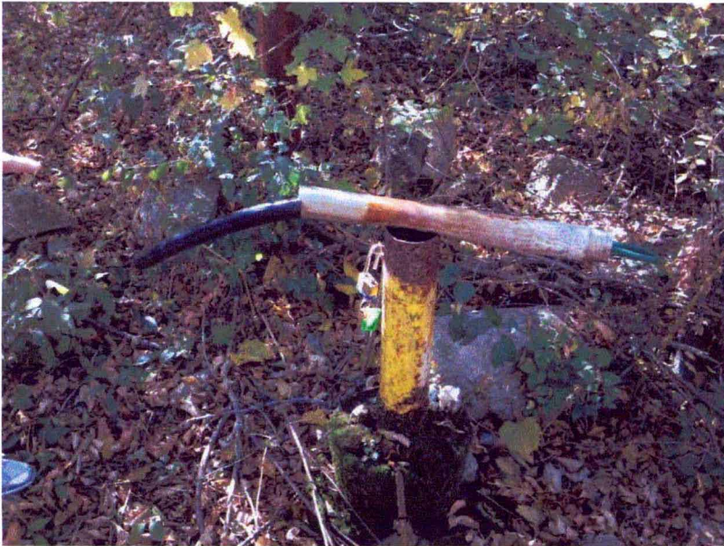
2012-10-017: MW-7B – Broken Well Casing
