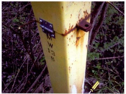
2013-014: MW-13S - New Hinge and Clasp Installed
