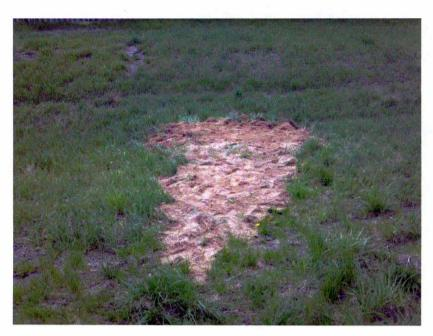
2013-001: Erosion Gulley Backfilled and Compacted
