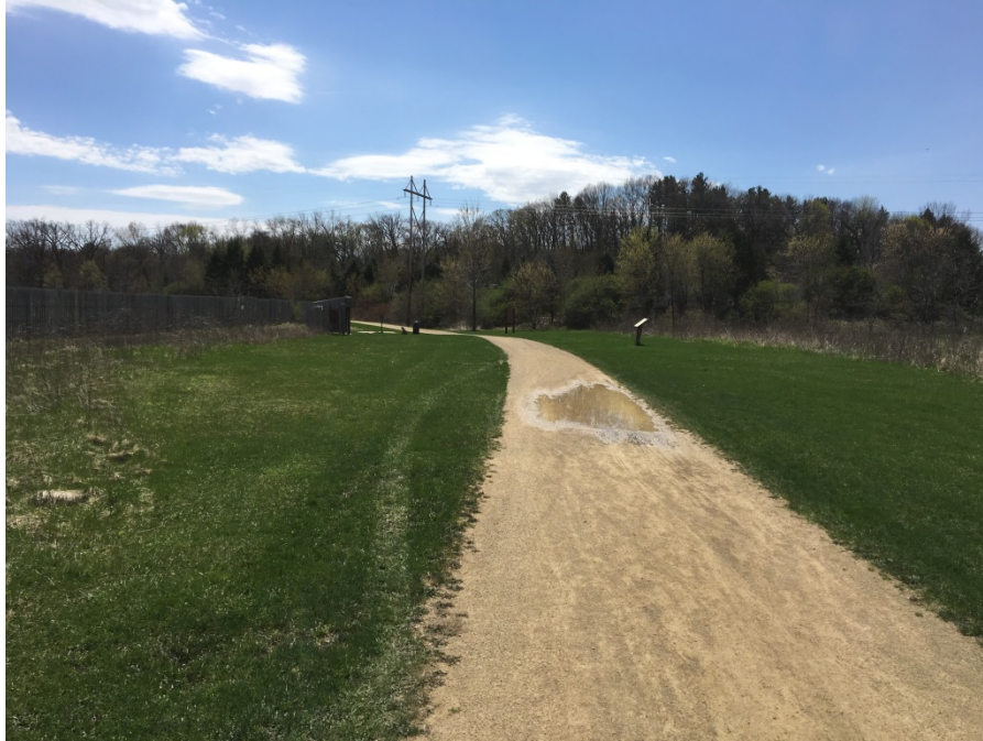
Photo 3: Photo facing south just outside the west access gate. Gravel drive around the west side of the landfill.
