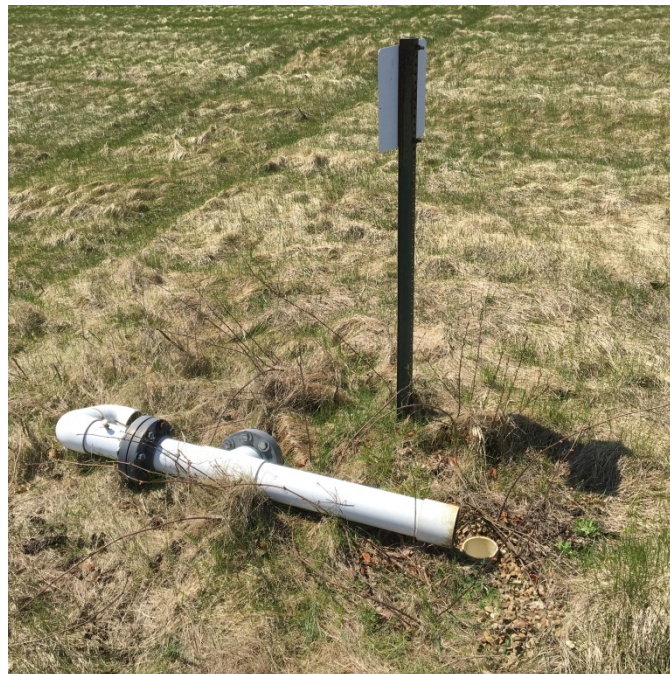
Photo 4: Photo facing northwest. Photo taken of GV-8.
