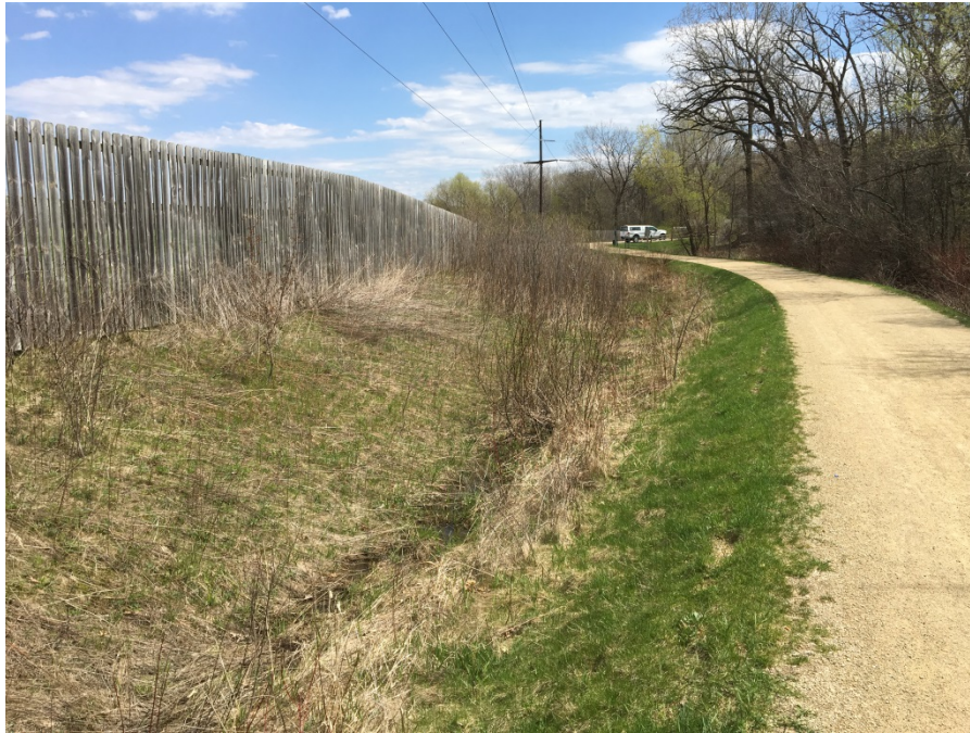
Photo 7: Photo facing east on the gravel drive south of the landfill. Site fence, storm water swale, and access road depicted above.
