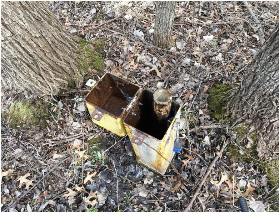
Photo 7: MW-10I casing flooded with water (looking down).
