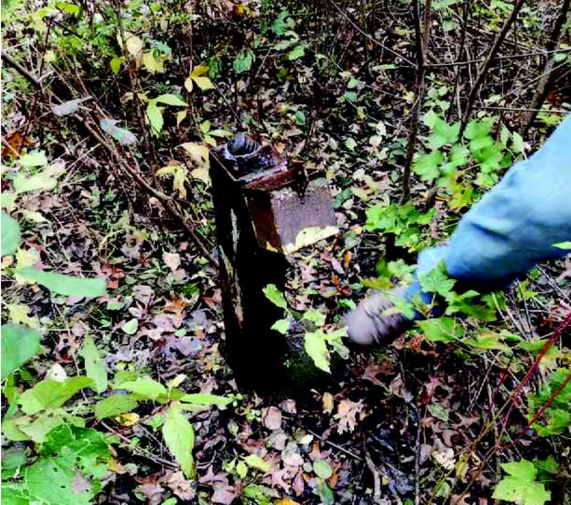
Photo 14: View toward monitoring well OW-02. Well is flowing and cap is floating on top of casing.
