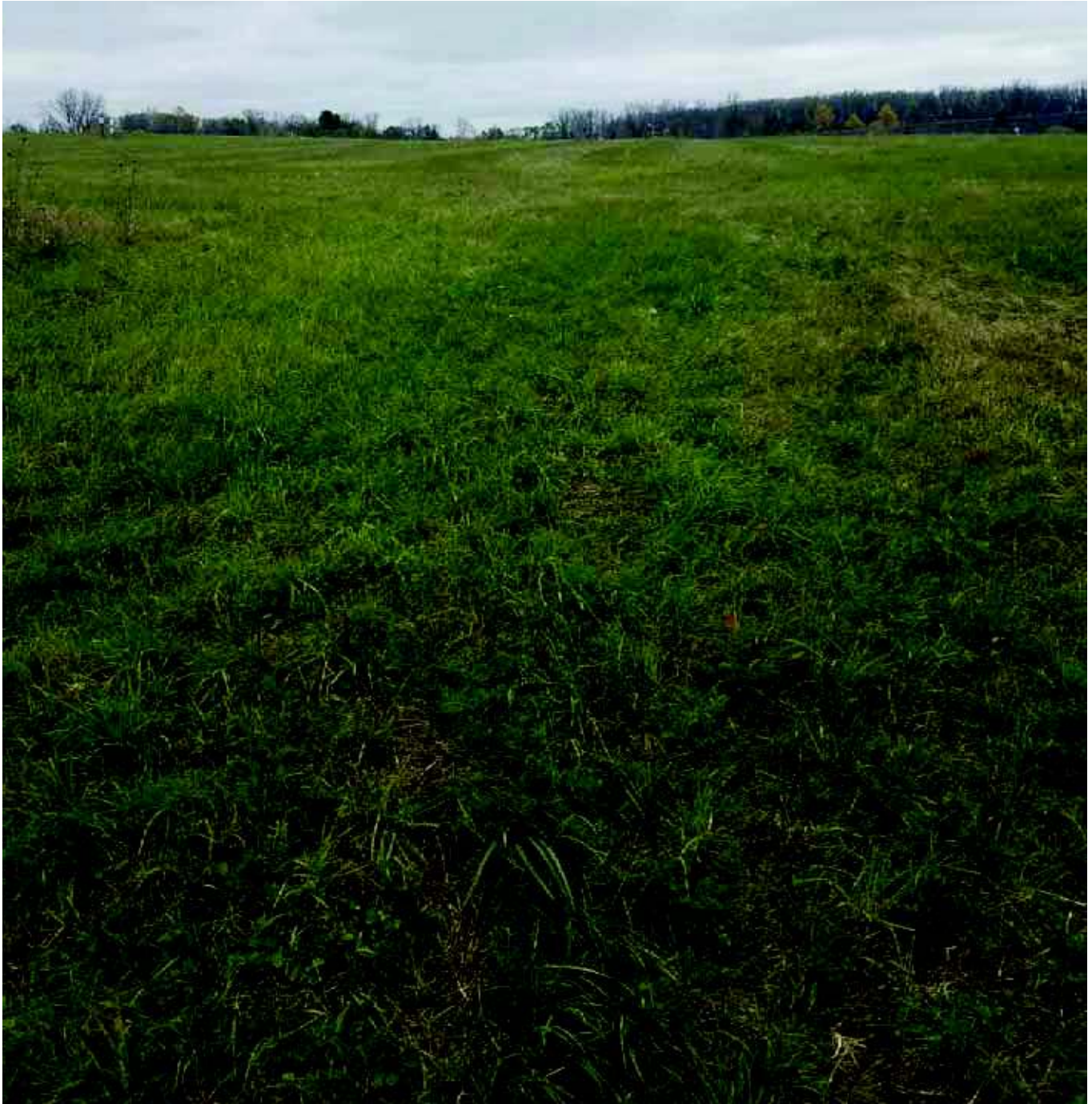
Photo 3: View north from south portion of site. Cap was in good condition.
