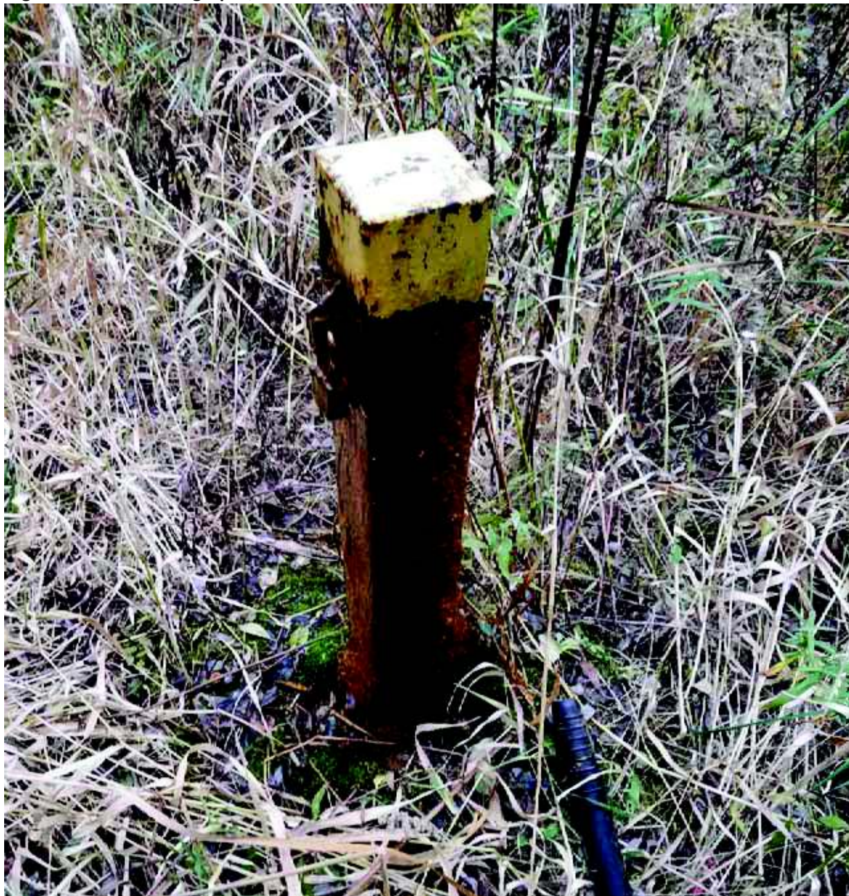
Photo 15: View toward monitoring well 131. Well is flowing and plug is on ground.
