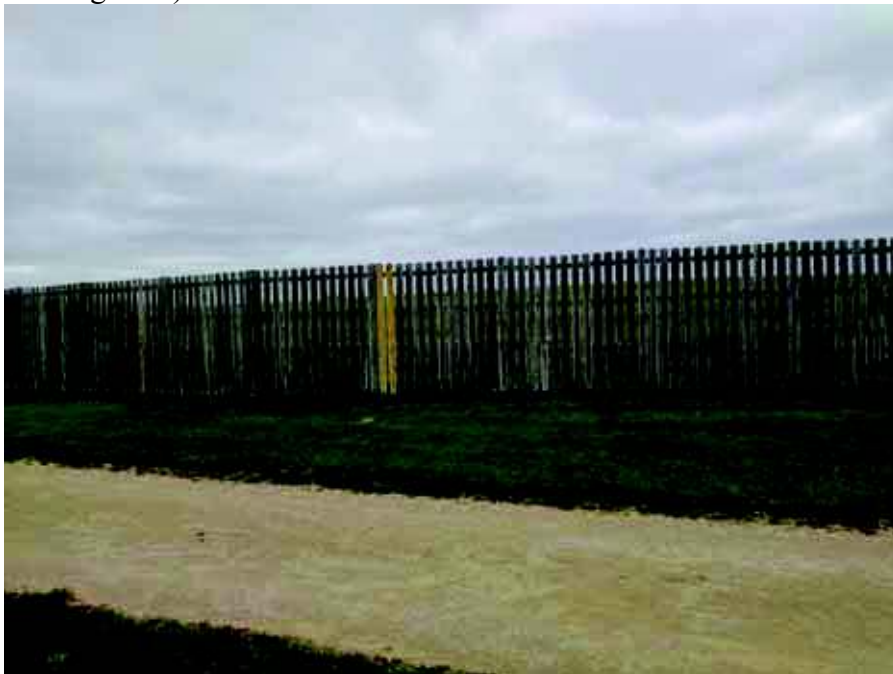
Photo 6: West perimeter security fencing depicted, slats were recently repaired (Looking east)
