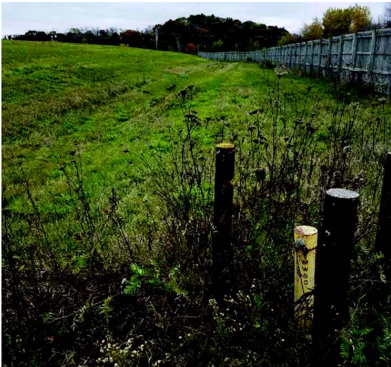
Photo 8: View south toward monitoring well MW-5D and storm water drainage along west edge of landfill.
