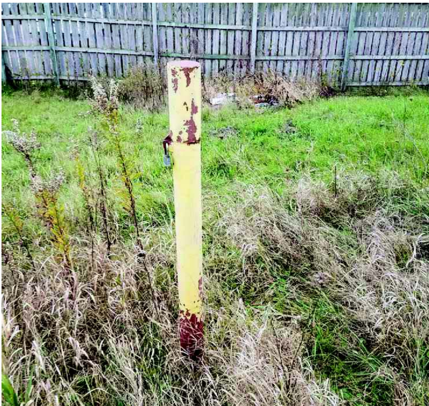
Photo 4: View toward monitoring well MW-2S. Several wells were not properly labeled.
