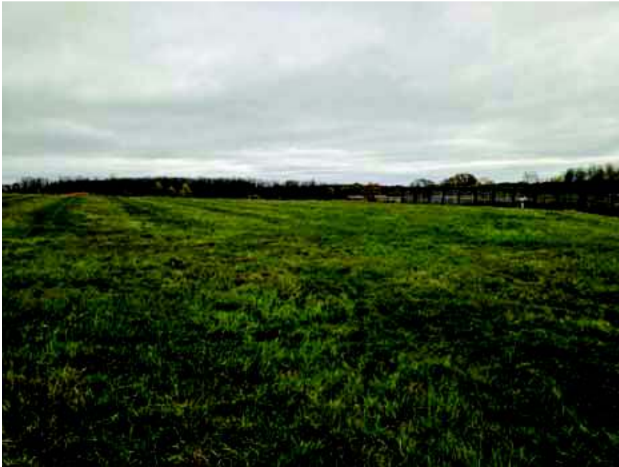
Photo 1: Photo taken just inside the south access gate. Final cover vegetation was in good condition and of the appropriate length (Looking north)
