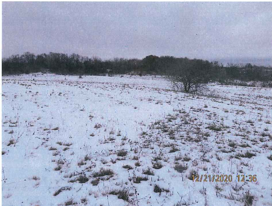
Photo 20: Minor area of settlement in northeast area of the landfill cap – view is to the north.
