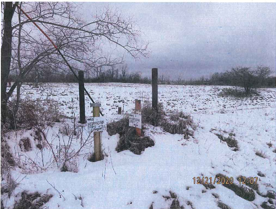
Photo 8: Groundwater Monitoring Well MW7 and LFAS point P7B.
