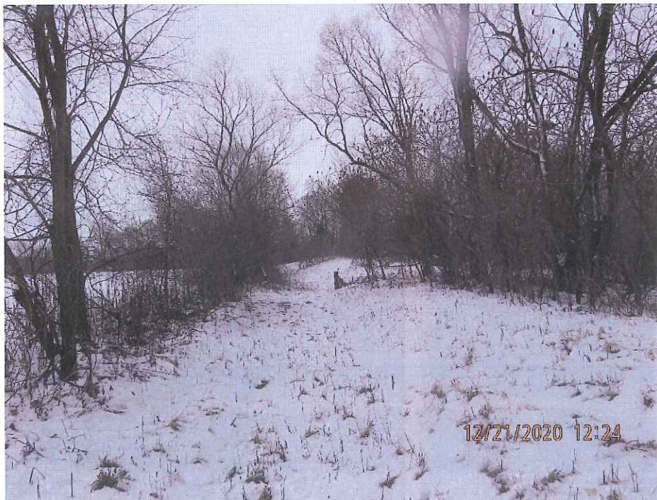
Photo 14: View looking to the south along the west perimeter of the landfill cap.
