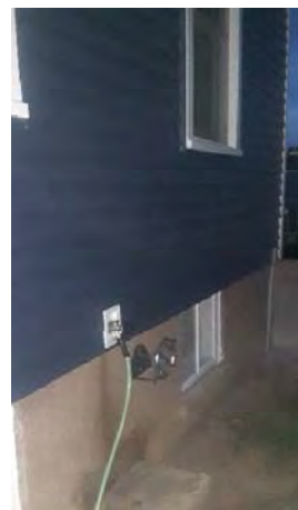
Photo #38 Private Well PW-05 (2611 County Highway O)
