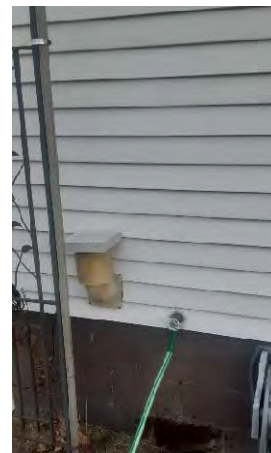
Photo #28 Private Well PW-07 (W2602 Elm St.)
