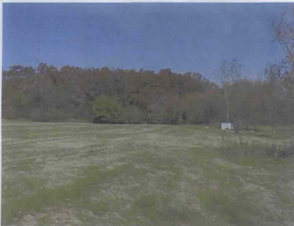
Photo 12 Looking N towards gas venting equipment from E side of LF
