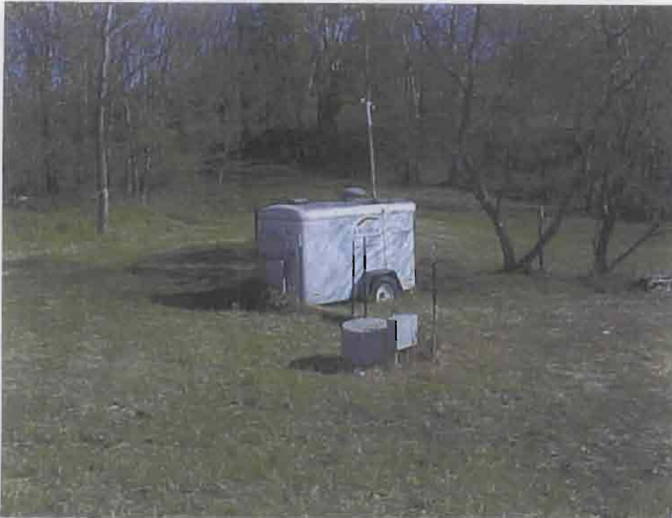
Photo 13 Active gas venting equipment; foreground drip tank, background is blower system trailer
