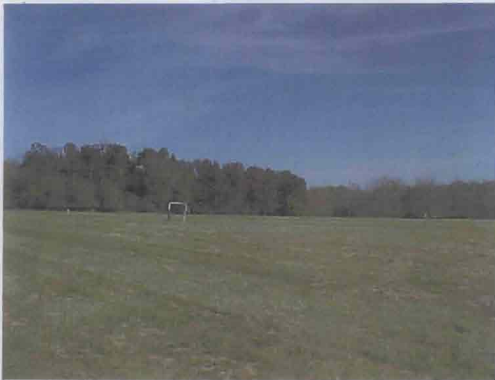
Photo 2 Looking NE onto LF from SW corner; shows gas piping from leachate well LC-3
