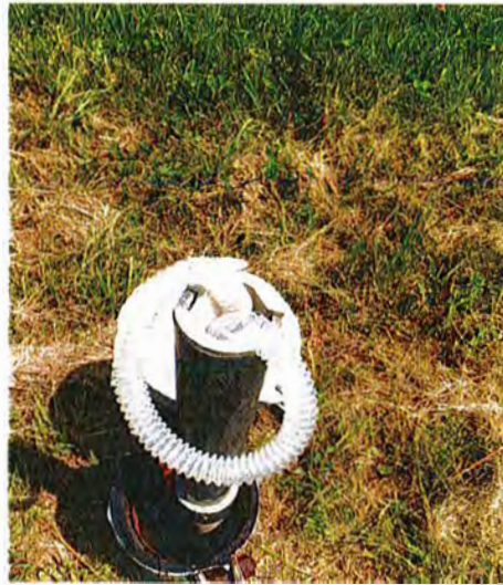
P-104, casing should be extended. It is damaging the well's discharge tubing.
